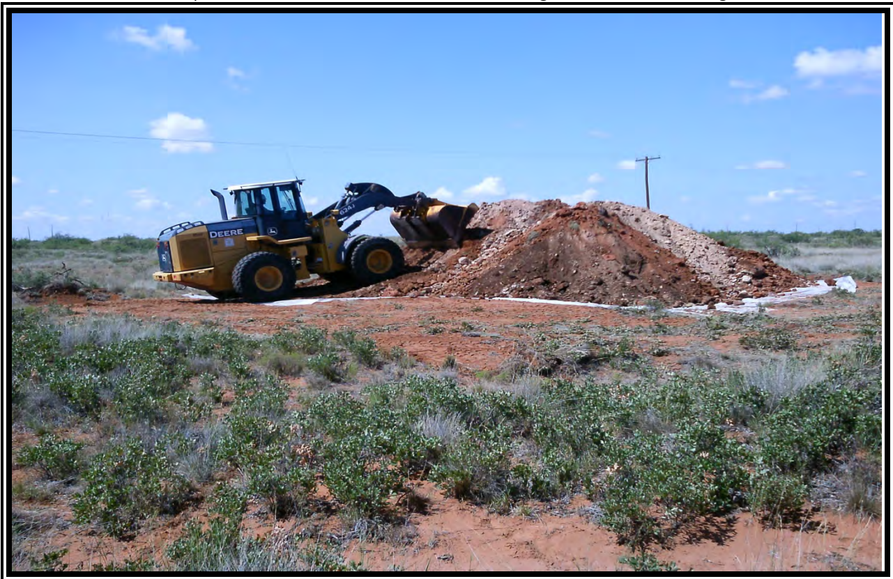
Placing excavated soils on plastic looking southwest.
