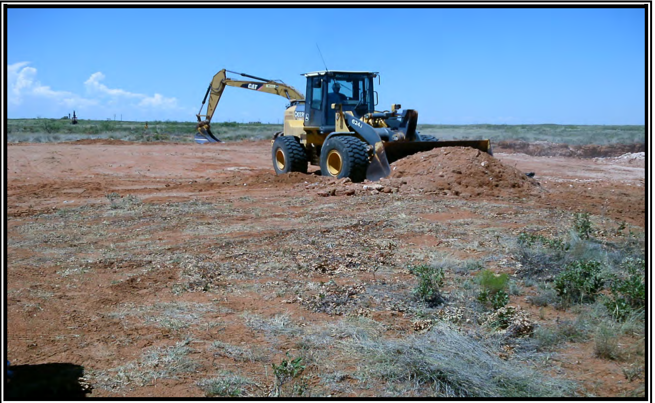
Picking up last of excavated soil for hauling to J&L Landfarm looking northwest.
