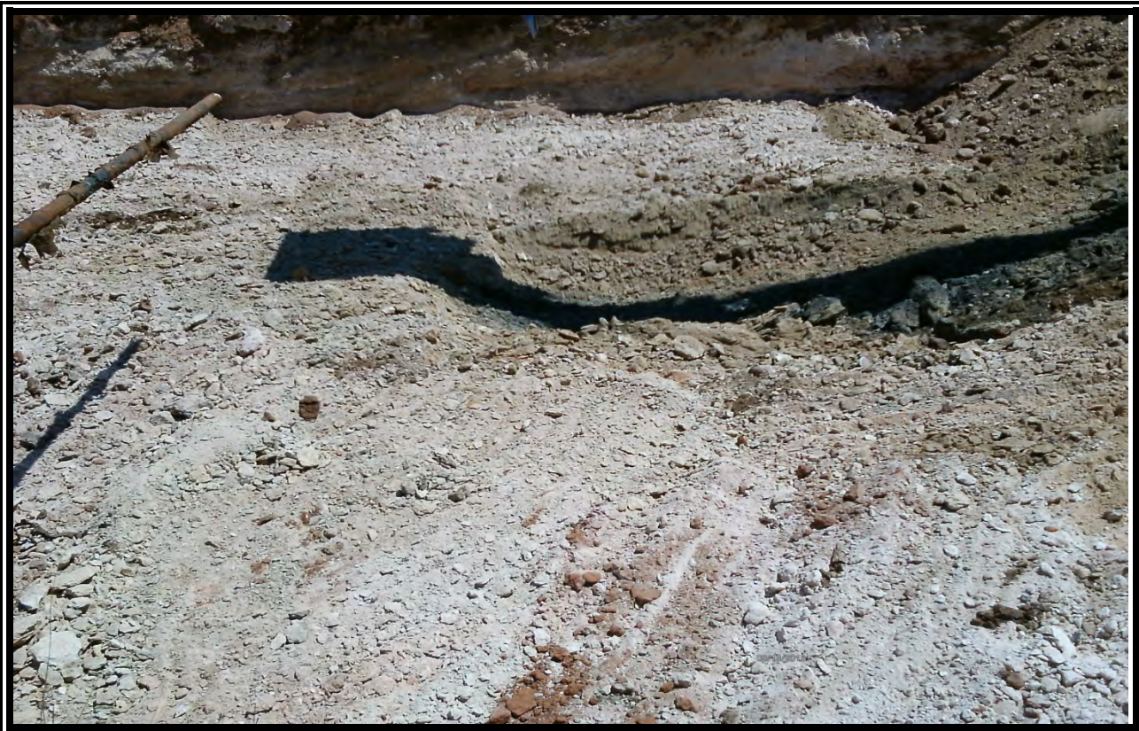
Discolored soils near end of 2" steel flow line looking south.
