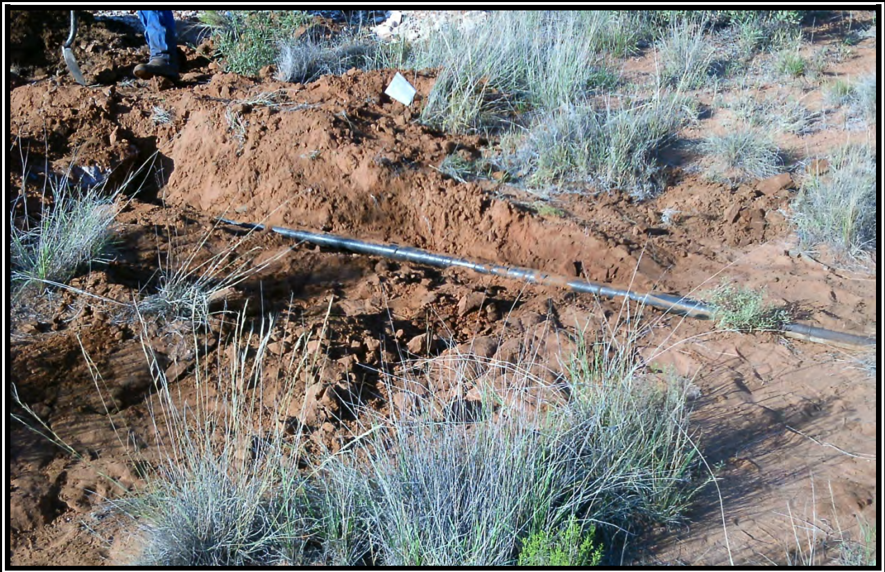
View of uncovering 2" steel flow line looking southwest.
