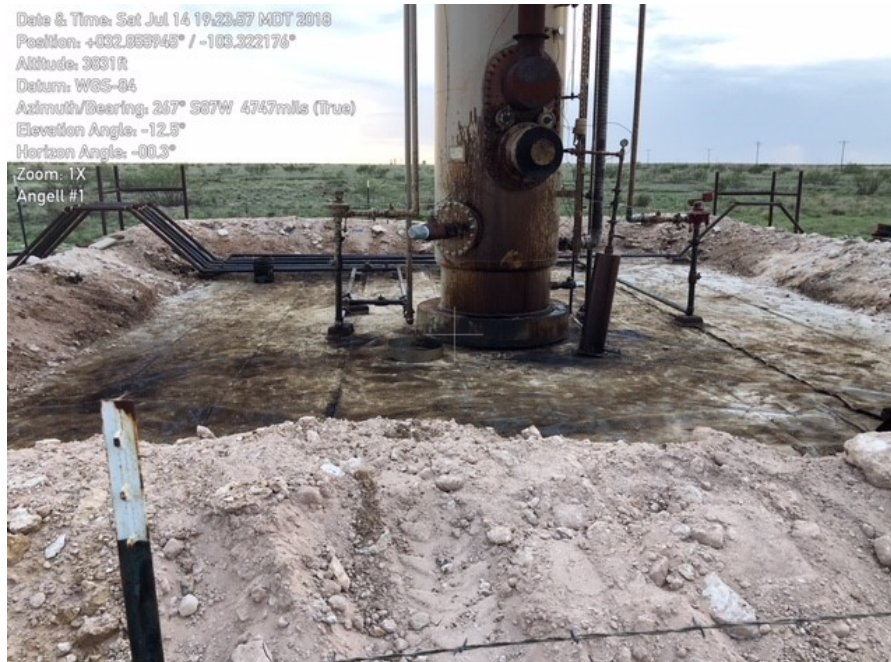
Photo 1. View of the secondary containment, liner after integrity inspection, looking west
