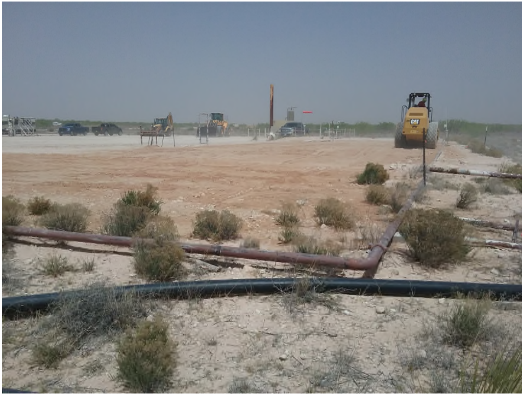
View North – Backfilled Excavation Area
