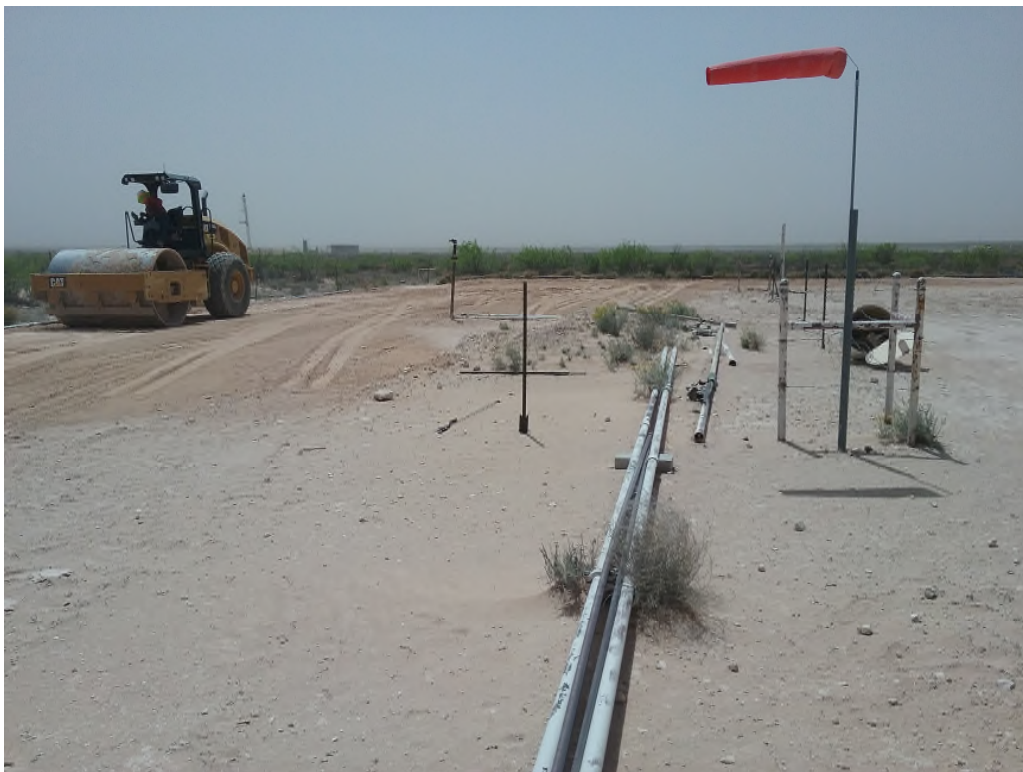
View South – Backfilled Excavation Area
