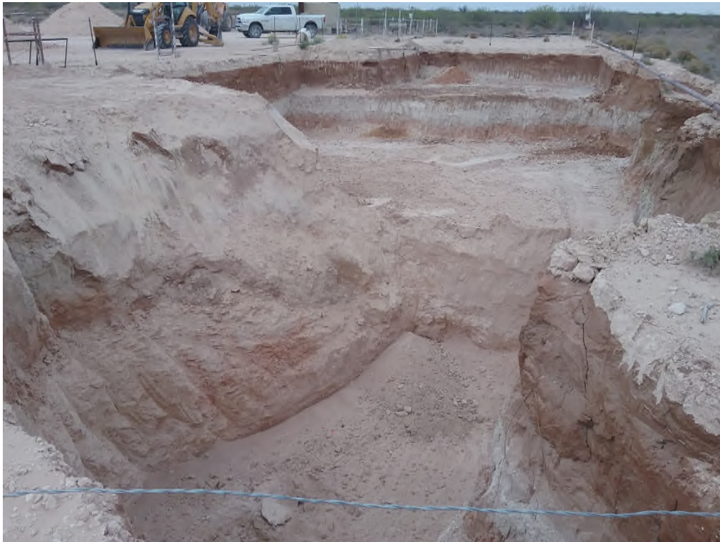
View North – Excavation Area
