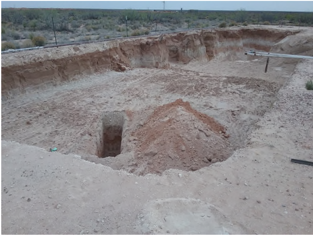
View South – Excavated area of BH-3
