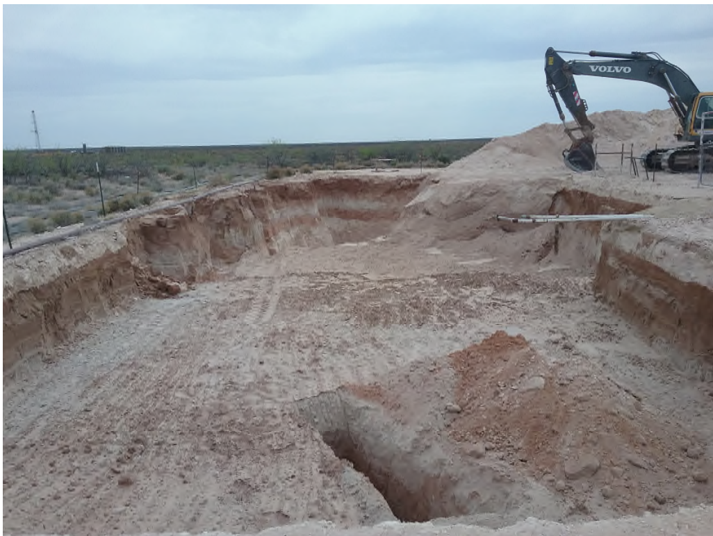
View South – Excavation Area
