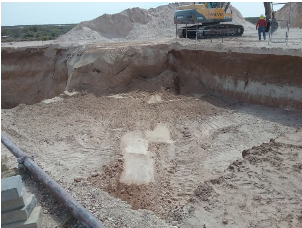
View South – Excavated Area of BH-2
