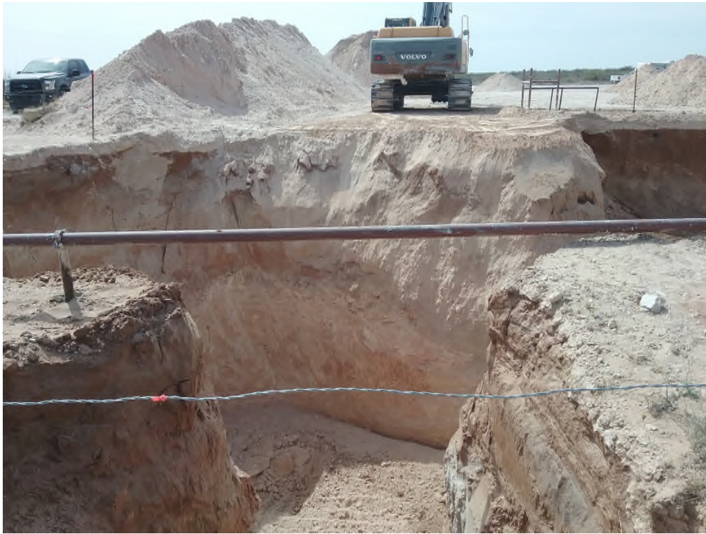
View West – Excavated Area of BH-1
