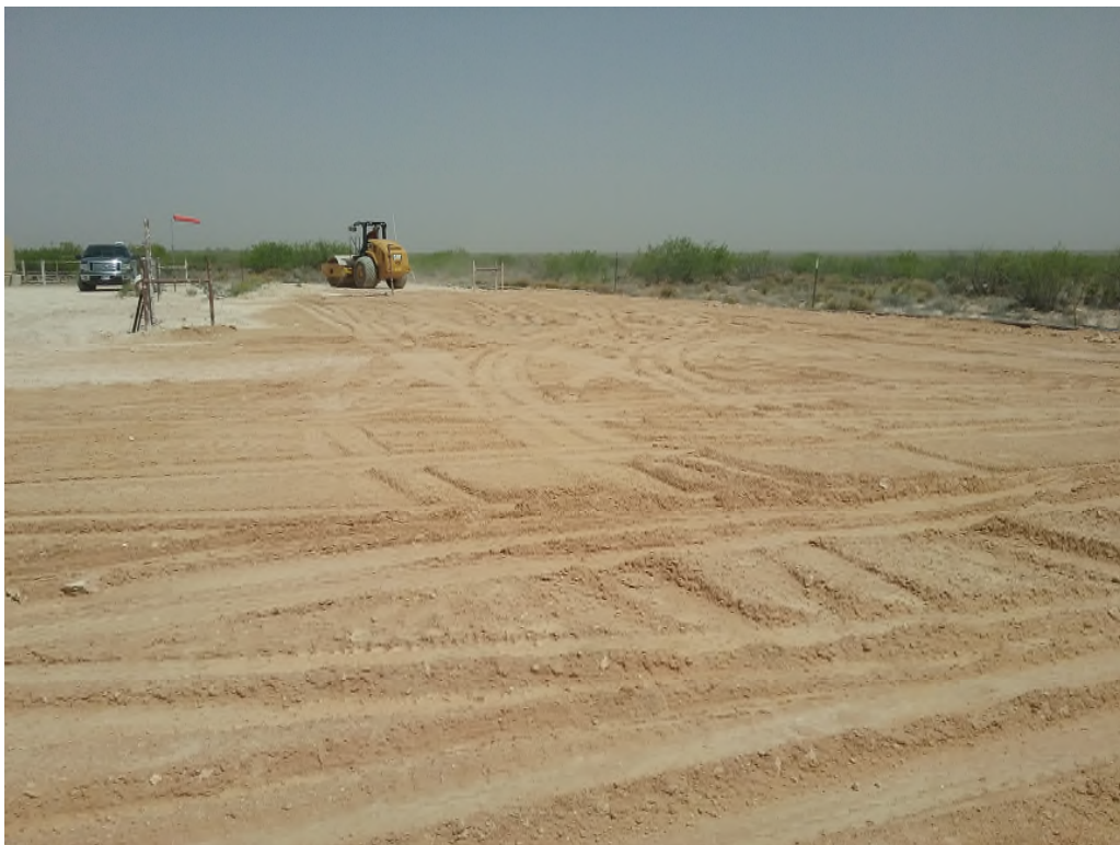
View North – Backfilled Excavation Area
