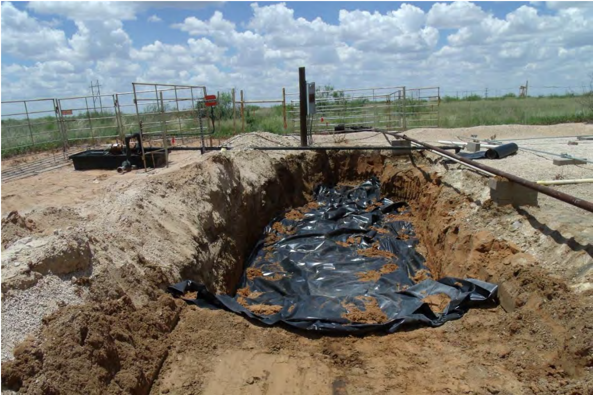
Photograph #6- Excavation and liner
