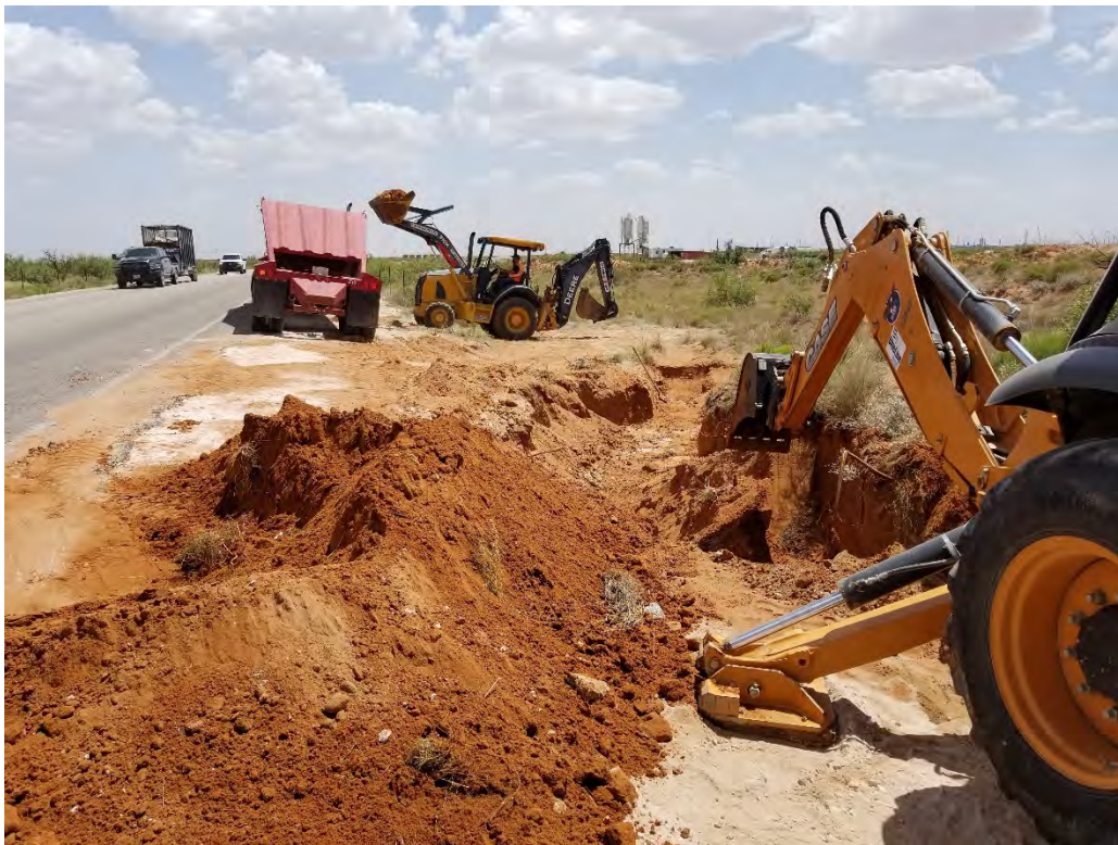
Photograph 4: View facing south, excavated soil being loaded for disposal
