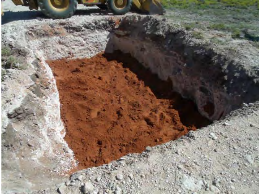
Photograph #13 Topsoil base on top of liner
