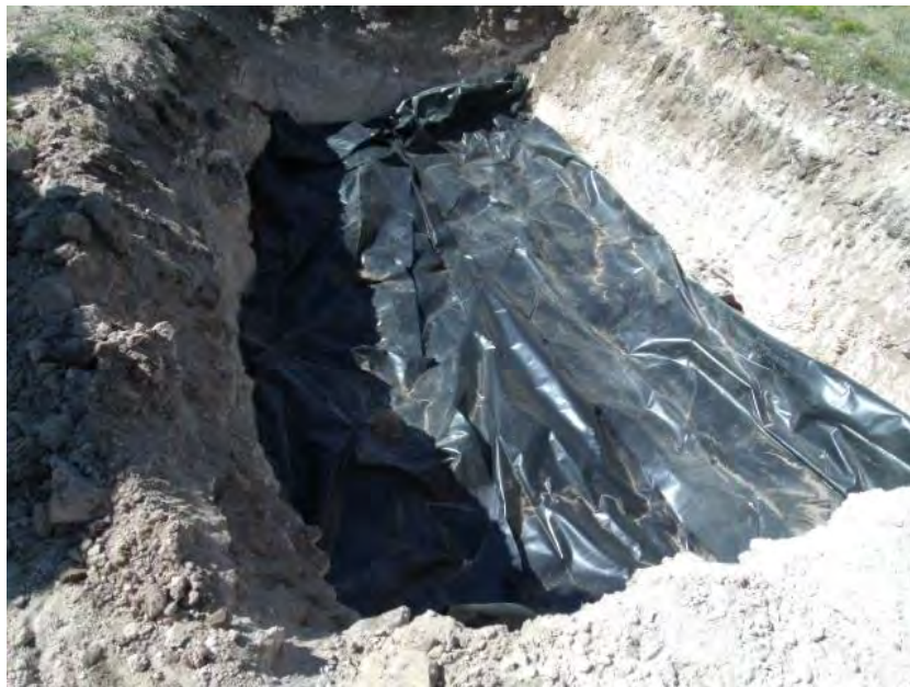
Photograph #12 Liner installed
