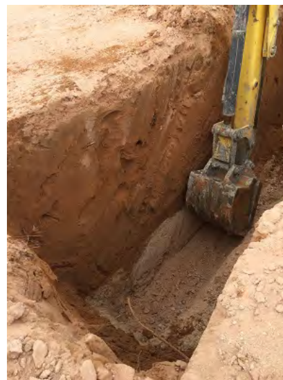
Exhibit B: Photo of lithology at Trench 2. Silty sand dominates the stratigraphic column from the surface to 5.5 feet. Very hard caliche was encountered at 5.5 feet.
