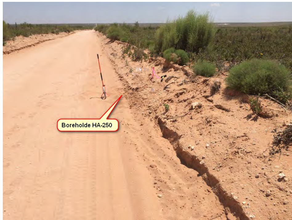
Figure M 7: Photo along BLM access road viewing south toward HA-250 borehole location. To drill at this location will involve grading the bar ditch and destroying vegetation. An arch clearance may be required prior to any grading activities.
