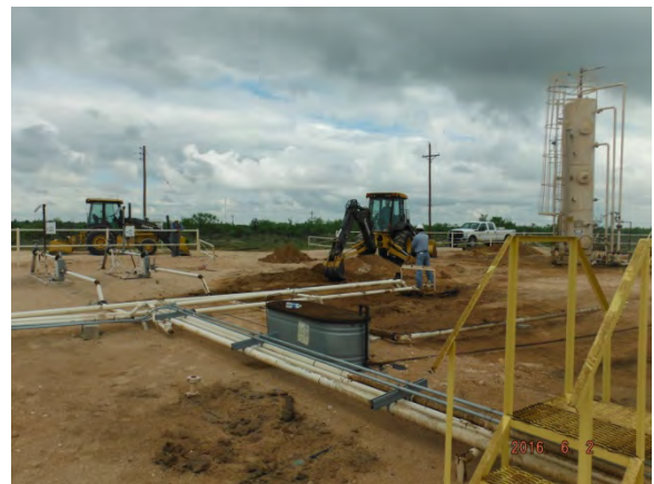
Excavating Leak Area, Facing NW 6/2/16
