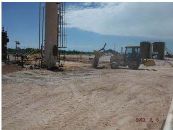
Backfilling Excavation, Facing SE 6/6/16
