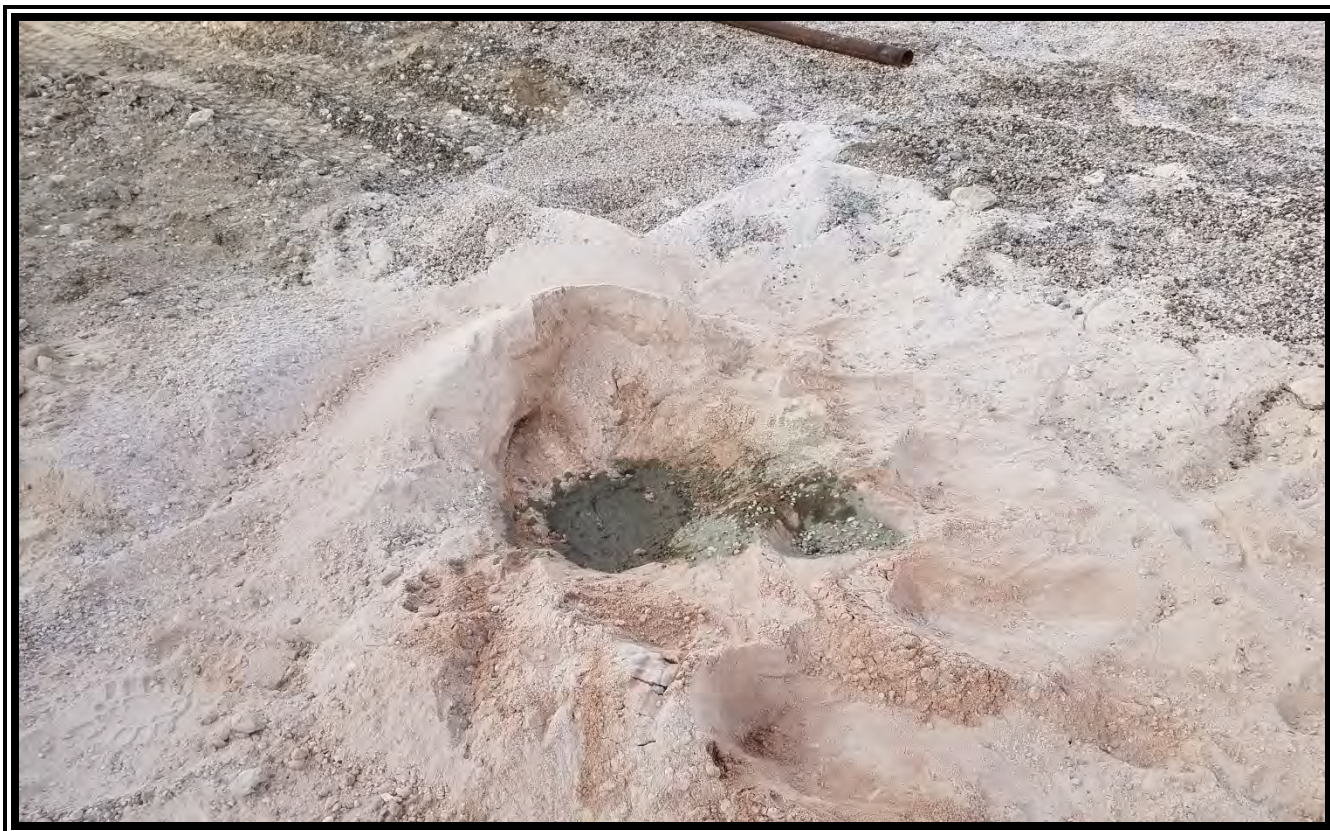
Close up view of boring Middle a after plugging and abandonment.
