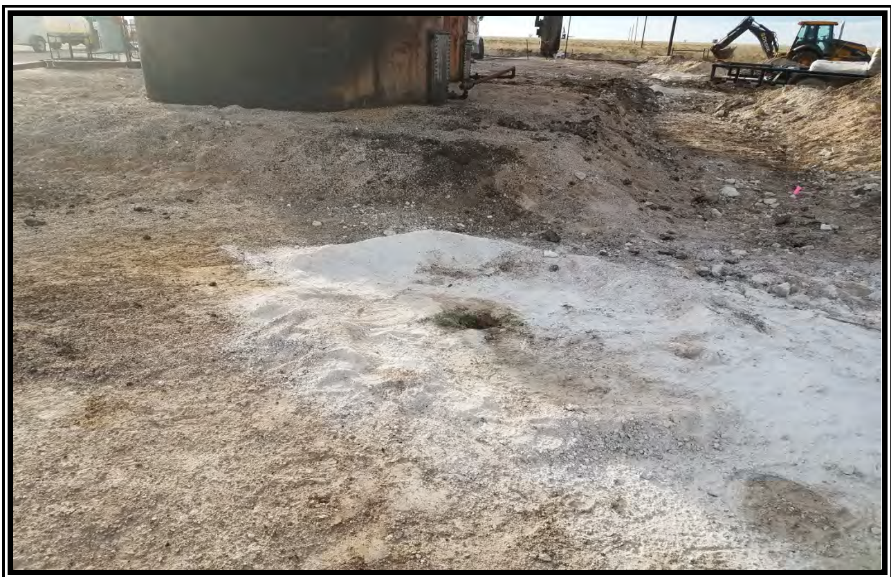
View of boring NE a after plugging and abandonment.
