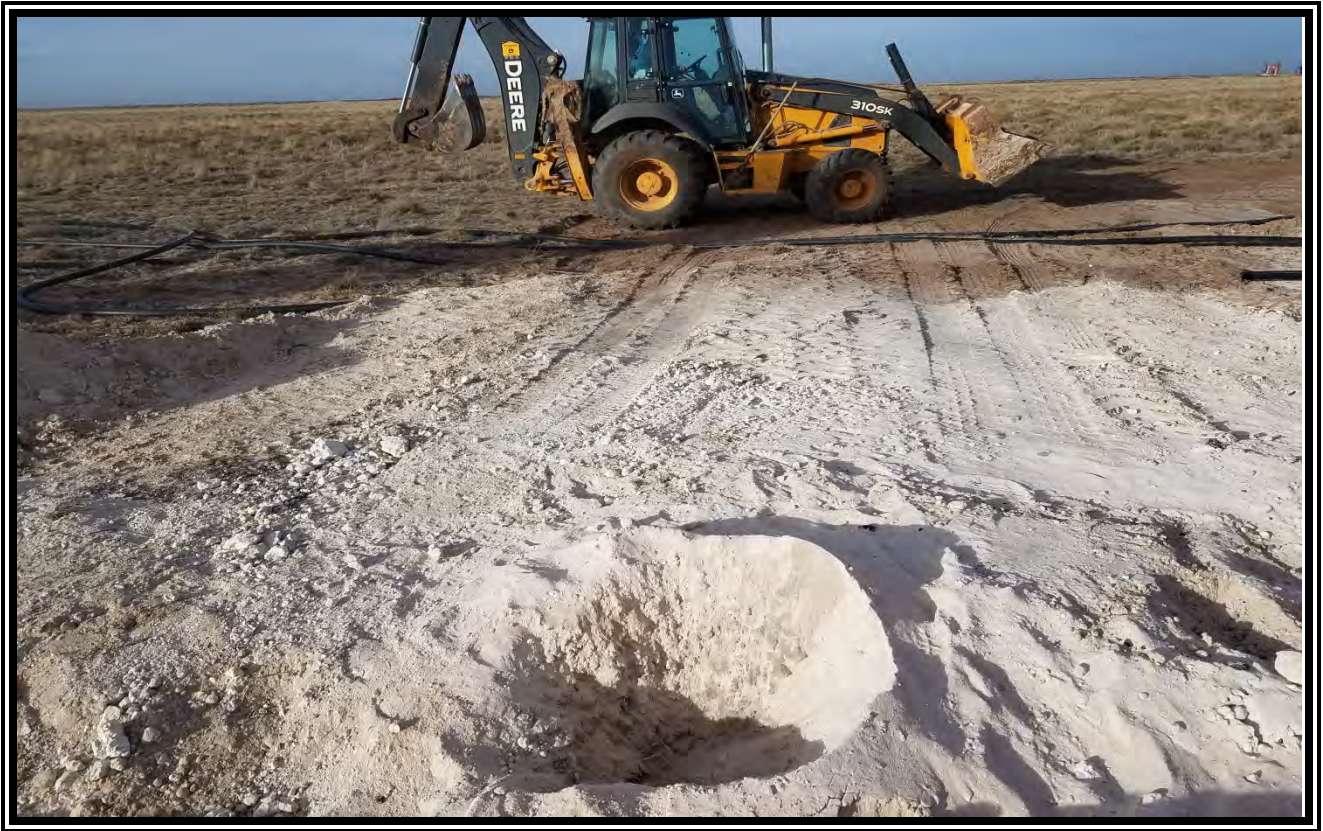
View of boring N2 after plugging and abandonment.
