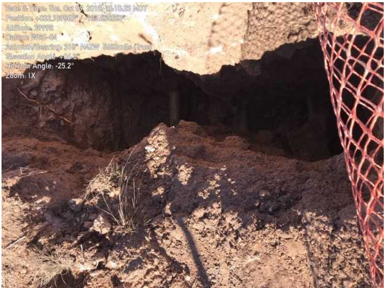
Photo 5: Hydroexcavated hole east of high pressure pipelines. Sample SW-9 location.
