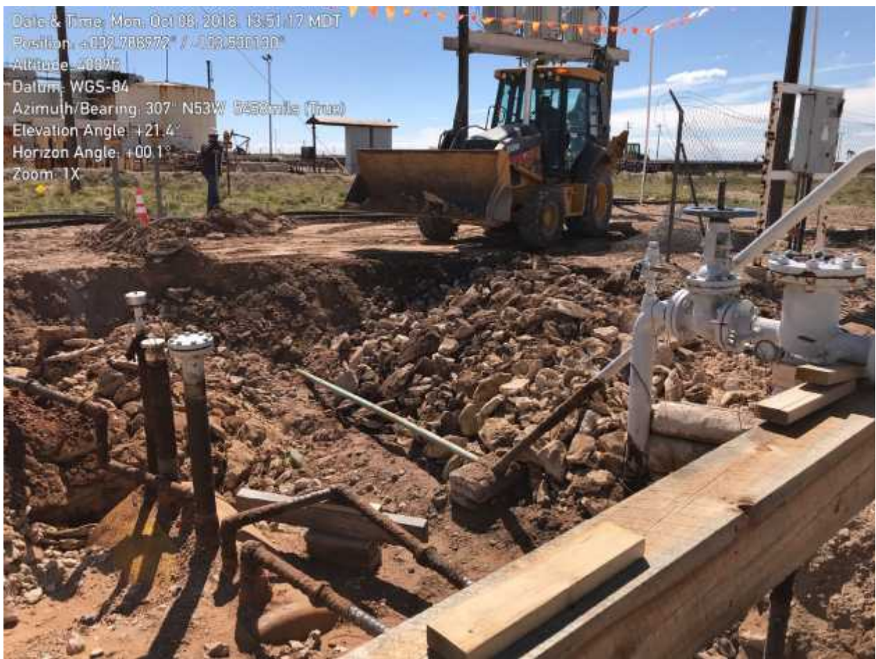
Photo 1: Additional excavation at sump/pipeline pumping unit.
