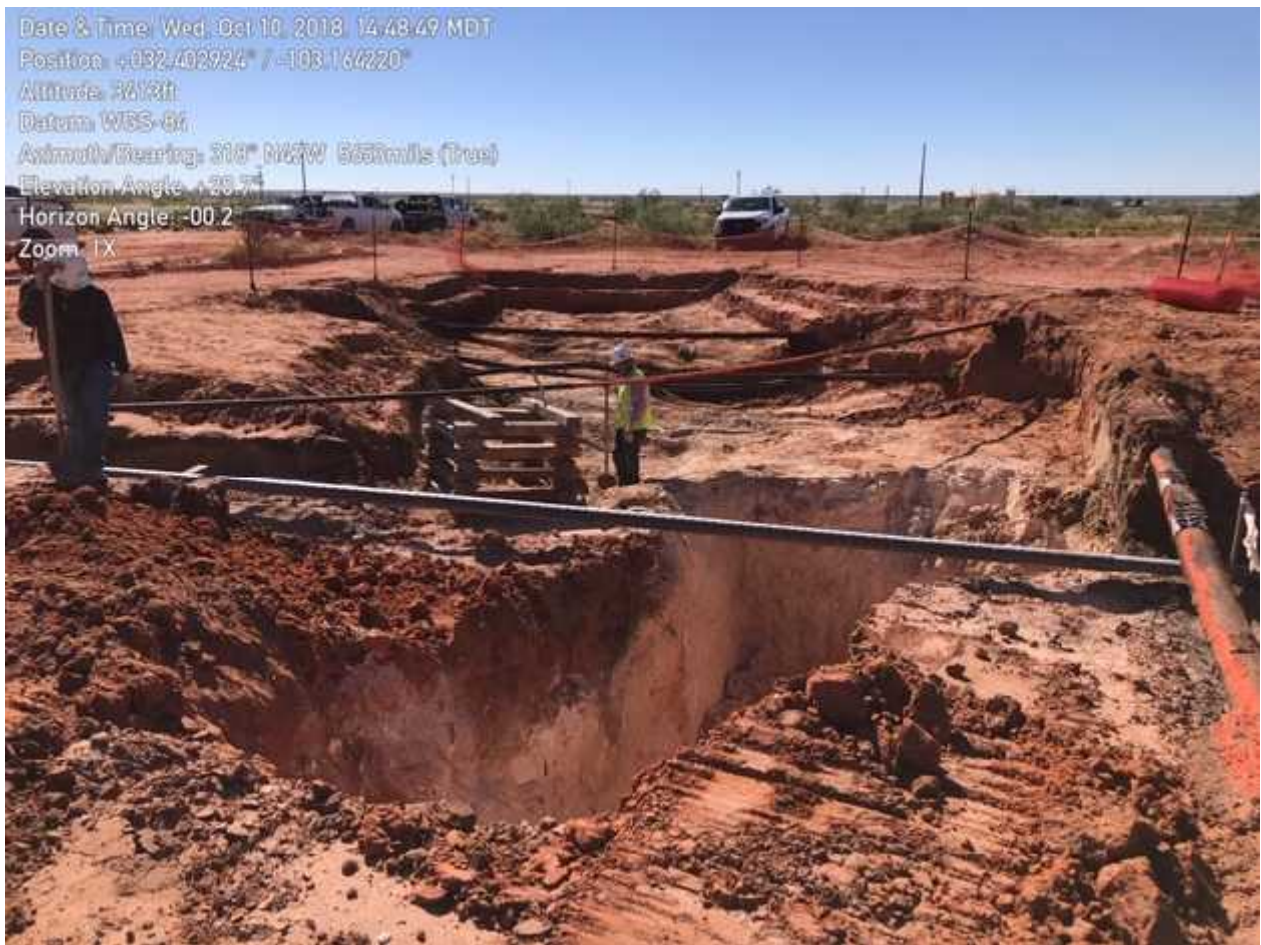
Photo 3: Trench beneath P66 crude line.
