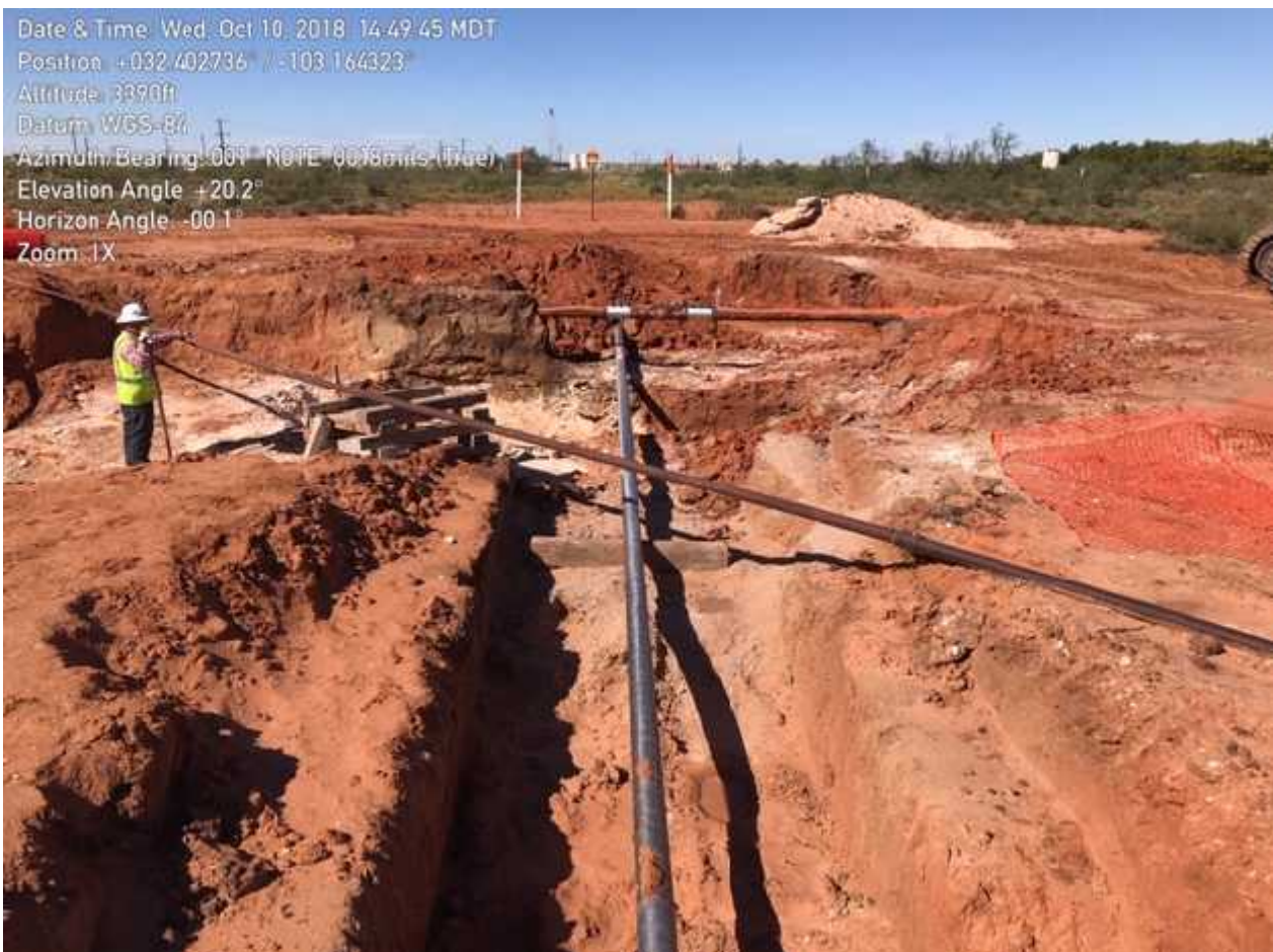
Photo 2: Surface flowline and repaired Targa pipeline overlying P66 crude pipeline. Rectangular excavated area in foreground not part of fresh crude impact excavation but rather to enable 40 ft P66 pipe joint replacement.
