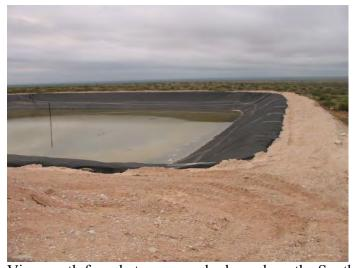
View south from between ponds shows how the South Pond levee is above natural grade.
