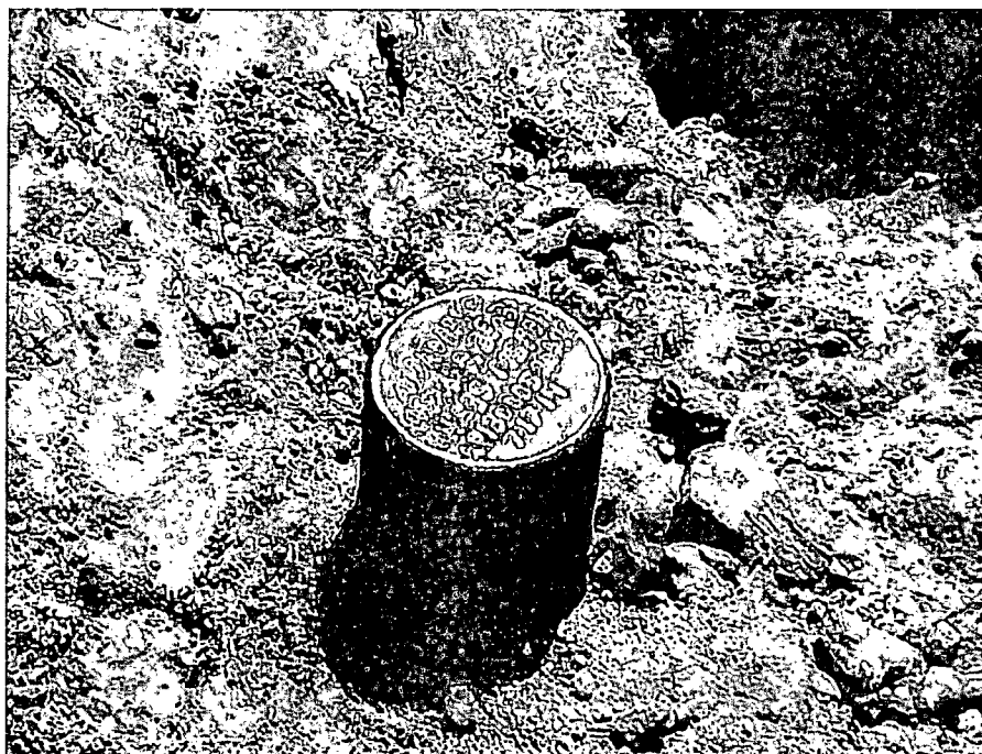
Photo 2 – Steel Well Cap Welded to the Top of the Surface Casing, four feet BGS.
