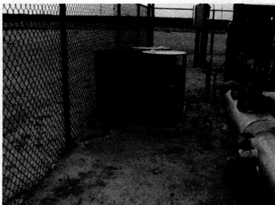
Drums of ethylene glycol stored on ground need to be on impermeable pad
