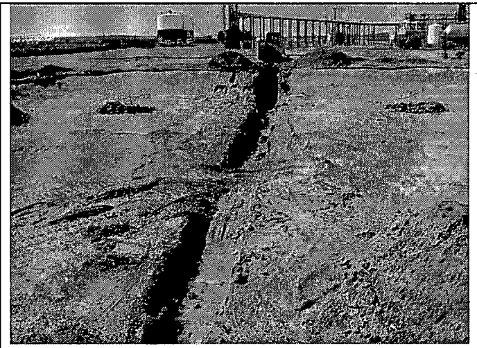
12.) Leak detection system removed from East Pond.
