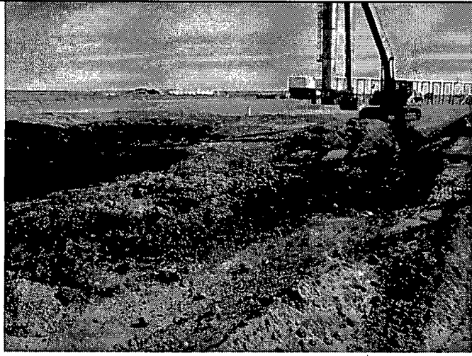
7.) Solidification of East Pond material utilizing blow sand.
