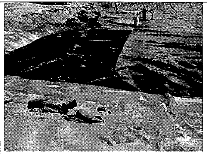
10.) Pressure washing and removing upper liner at East Pond.
