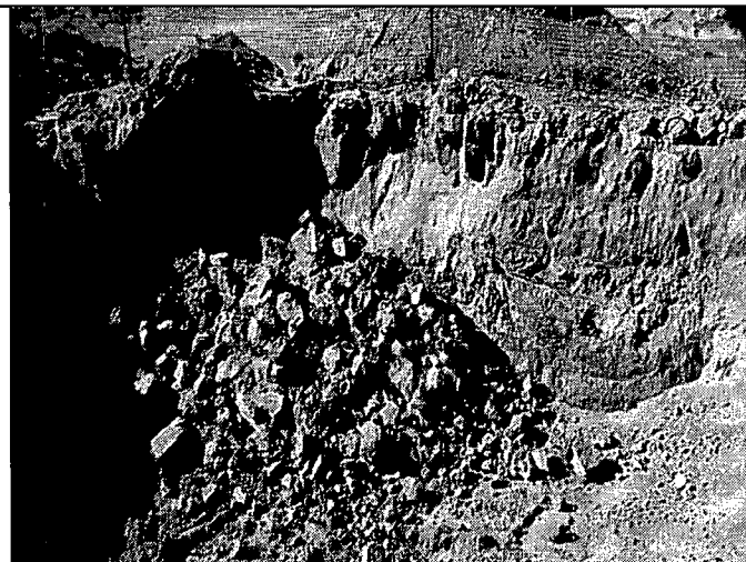
14.) General view of the over-excavation at south wall of East Pond. Minor slough occurred overnight. White/gray areas are clays.
