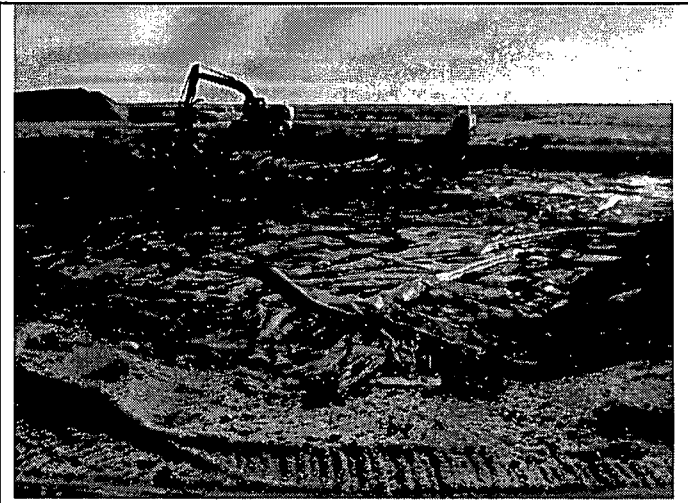
8.) Removal of solidified material in East Pond.
