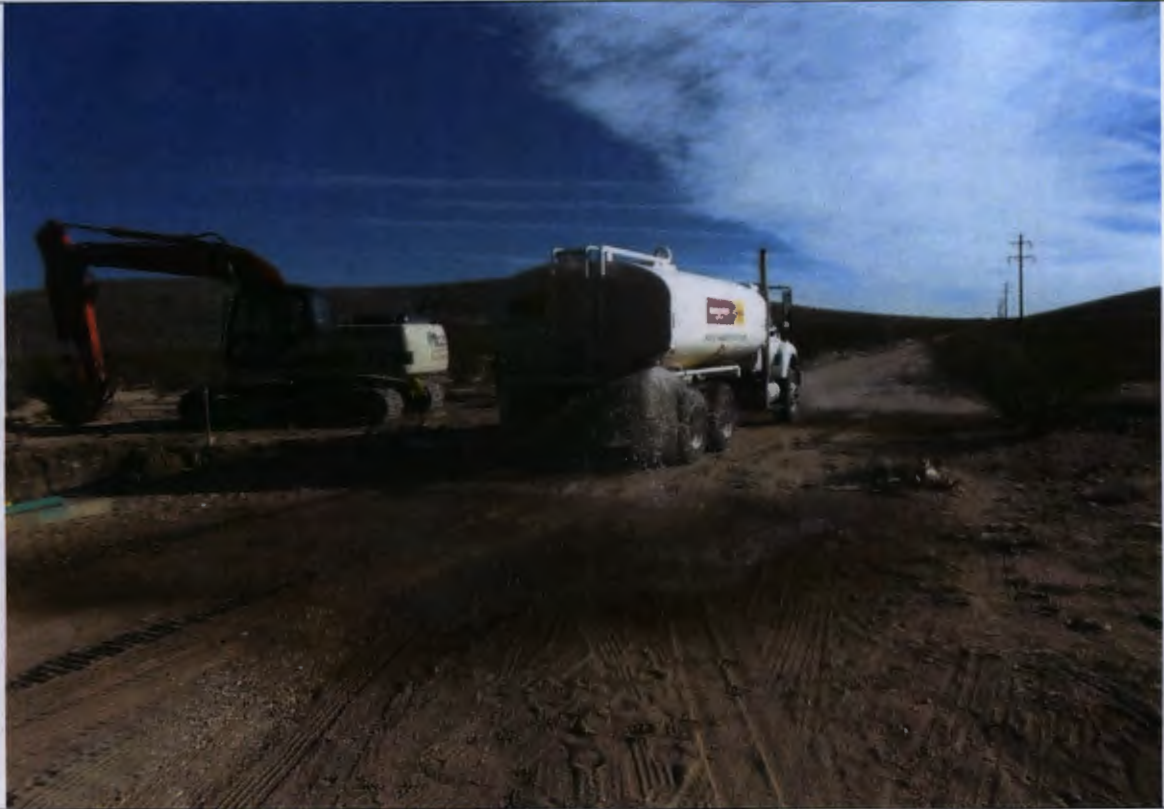
Photo No: 1 – RAD#13-0106 - EPNG Line No. 1005 Pipe Replacement Project Location: Section 17, Township 26 South, Range 17 West, Hidalgo County, New Mexico Comments: Photo of discharge used for dust control on the ROW.
