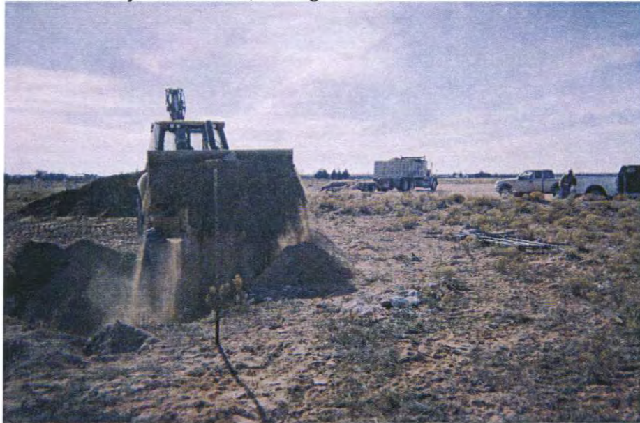
backfilling excavation with clean, imported soil in background, facing southwest
