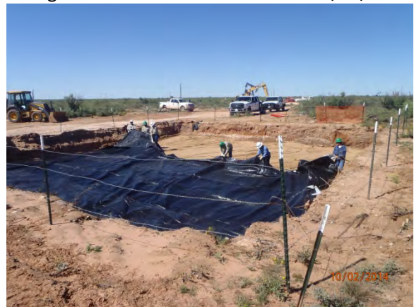
Installing 20-mil liner at 4.5 ft gs, facing northwest 10/2/2014
