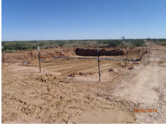
47x48-ft liner installed with 6 inch top soil pad, facing southeast 10/2/2014
