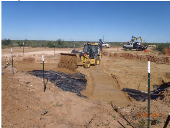
Padding above the liner with 6 inches of top soil, facing north west 10/3/2014
