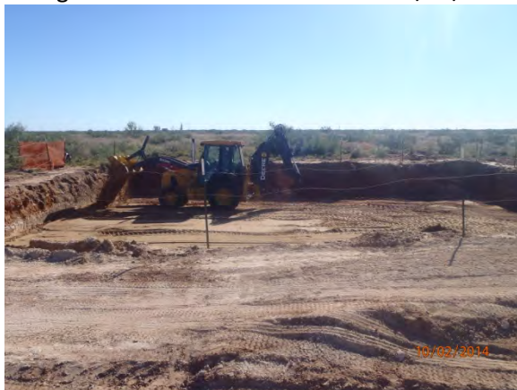
Padding excavation with 6" of topsoil, facing east 10/2/2014
