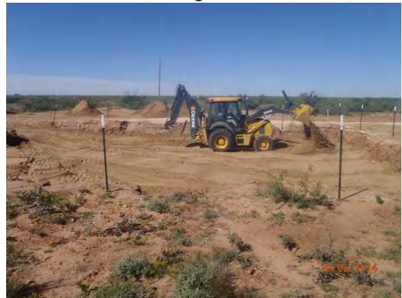
Backfilling above liner, facing west 10/6/2014
