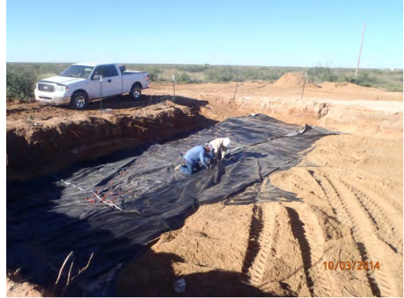
Installing and seaming the 47x12-ft liner with the 47x48-ft liner, facing southwest 10/3/2014
