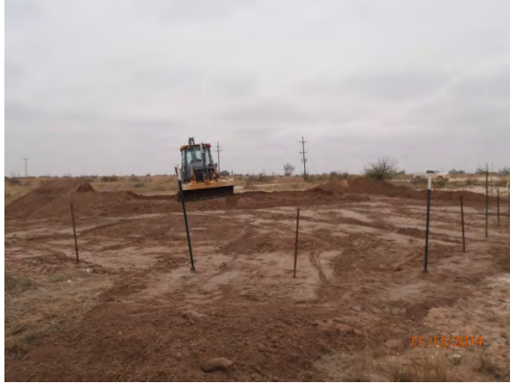
Spreading topsoil, facing northwest 11/11/2013
