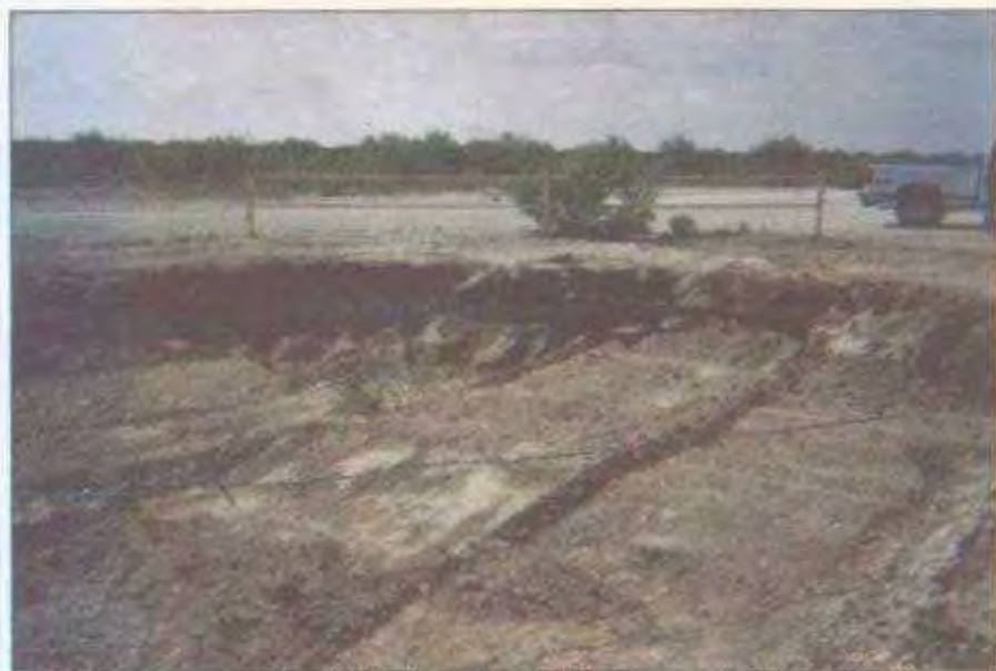
Excavation Backfilled to 4 ft With Remediated Backfill
