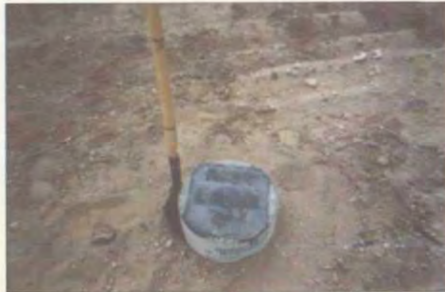
ID Plate Marking Clay Liner At Backfilled Site
