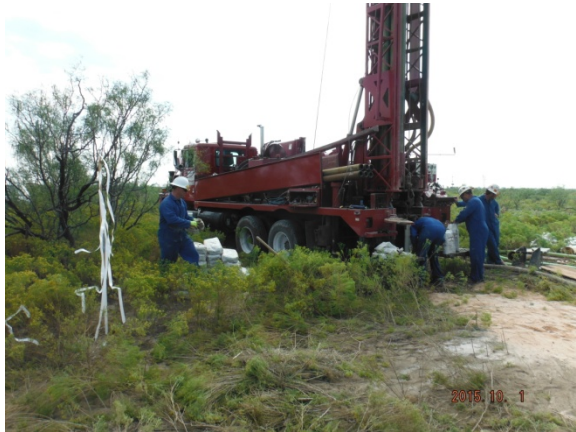
Adding the sand pack and bentonite seal 10/2/2015
