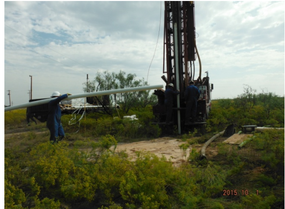
Installing casing in MW-3, facing northeast 10/2/2015
