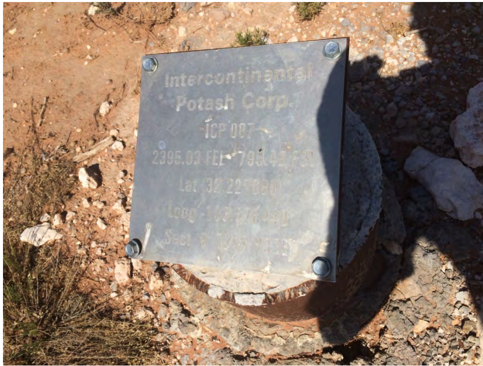
Photo 11: View of plugged casing of OSE well C-03565 POD 5; 2,500-feet northeast of AST.
