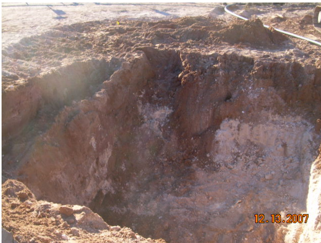
Photograph No. 6 – Looking southerly excavation II.
