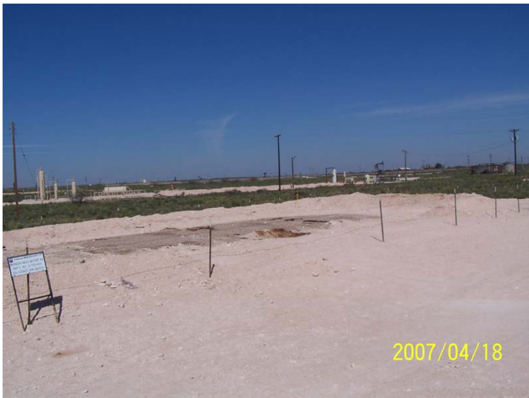
Photograph No. 2 – Looking northwest at tank battery bermed area (north end).
