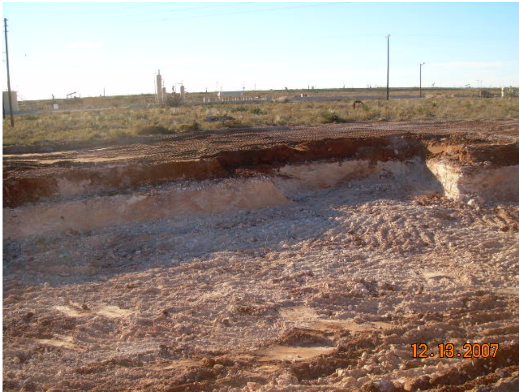
Photograph No. 5 – Looking westerly across Excavation II.
