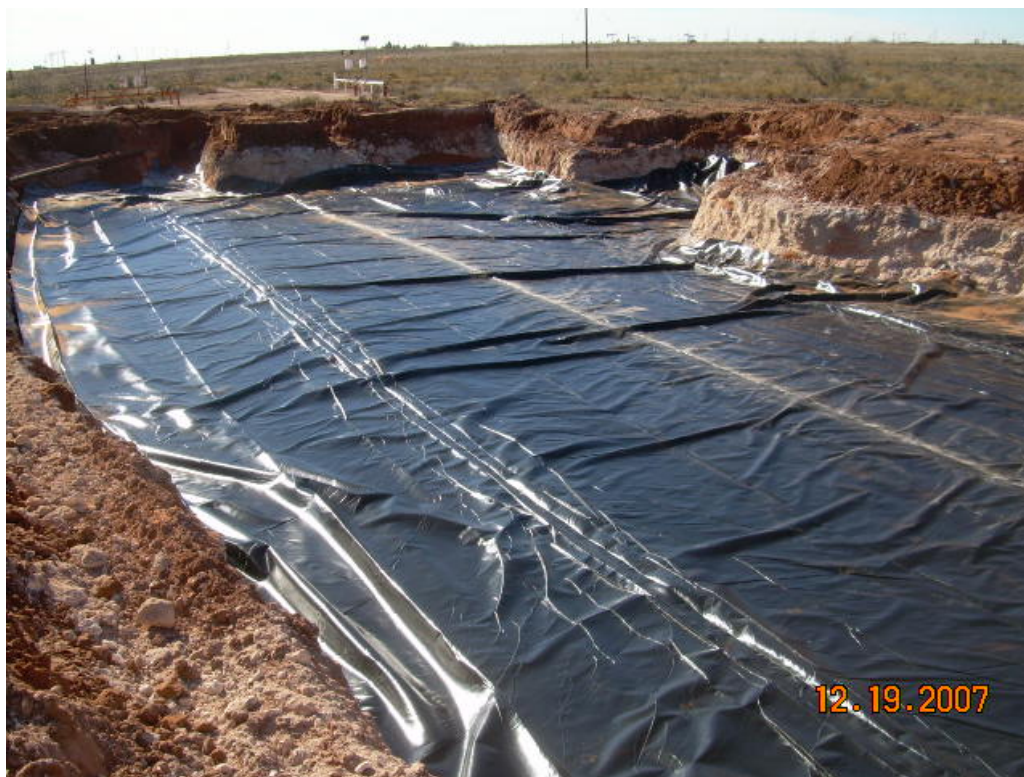
Photograph No. 8 – Looking southwest across Excavation I and installation of liner.
