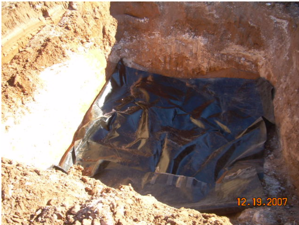
Photograph No. 9 – Looking southerly across excavation II and installation of liner.
