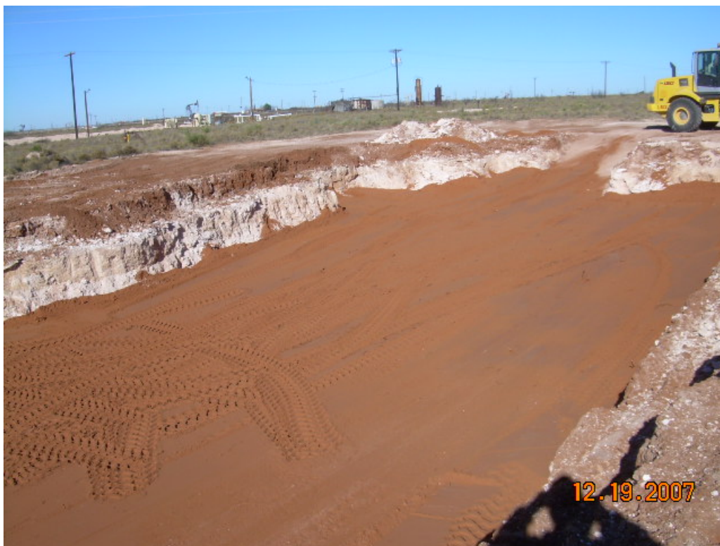
Photograph No. 7 – Looking northwesterly across excavation I with cushion material.
