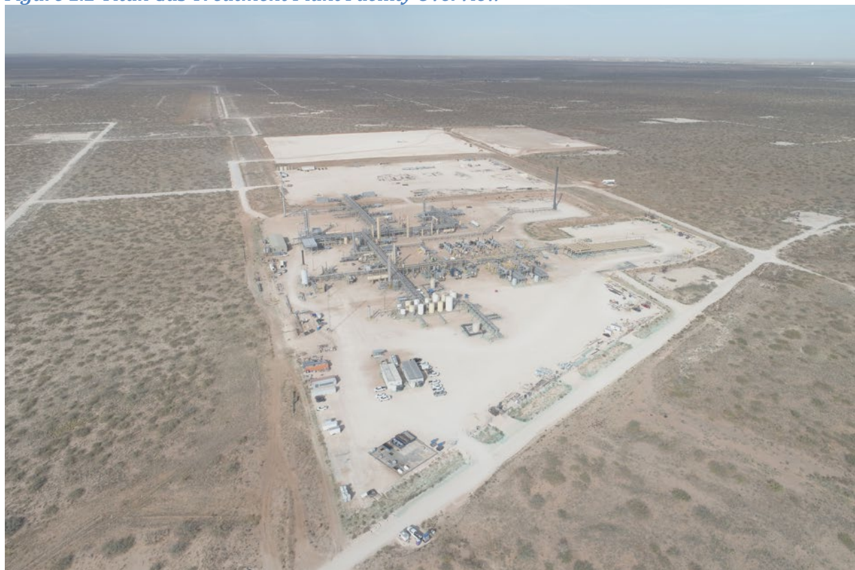
Figure 1.2 Titan Gas Treatment Plant Facility Overview
