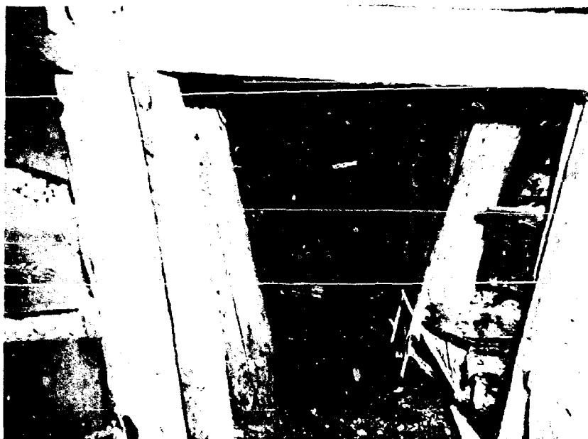
Figure 6.6. Postshot Timber Failure in Stope Area of Sheelite Mine.
