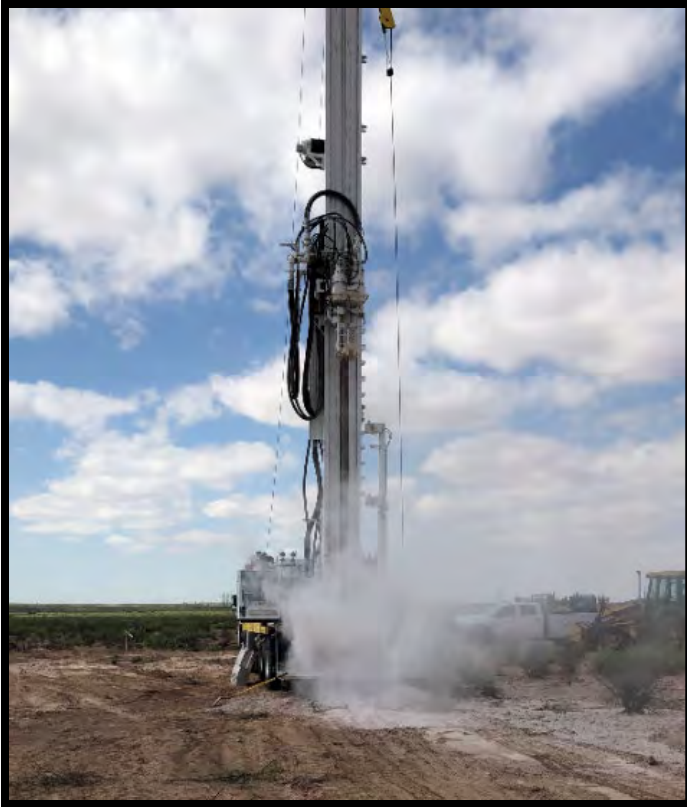
Image 1 - Drilling through dry gypsiferous soils.
