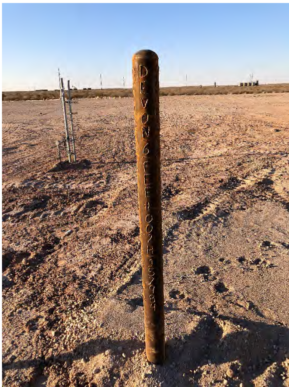
SP-1 View to north showing plugged well marker for Devon 6 Fee 2H. The Scout AST location is this former production pad.
