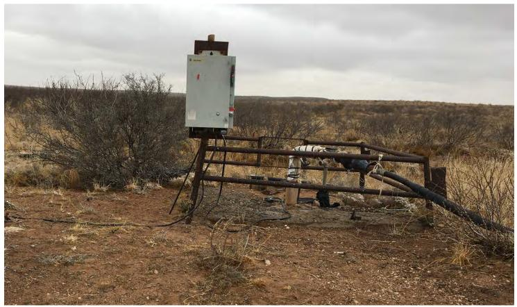
Figure SP8 – View north of pumping well (Misc-297) and plugged casing to the right of the steel fence (Misc-295). USGS data suggest that the pumping well was gauged by the USGS in 2013 and the data recorded as well USGS 14778 (see Figure 2a and 2c) but gauging data from 1965-1971 from the plugged well (Misc-295) was also recorded as USGS-14778. The mis-location and mixed gauging results in the USGS database are explained in the text of this submission.
