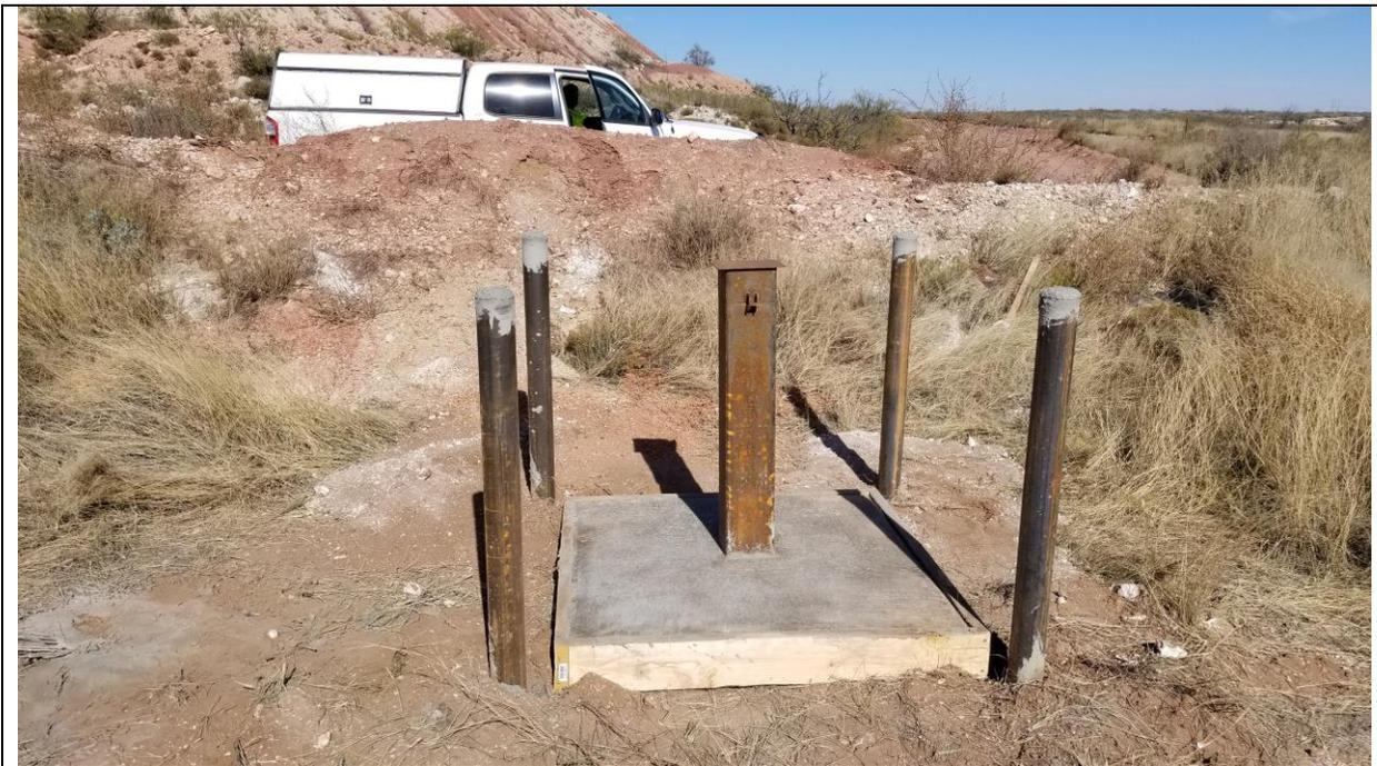
Photo 62—Surface completion, well VZ-2, OSE well permit no. CP-1692-POD-1
