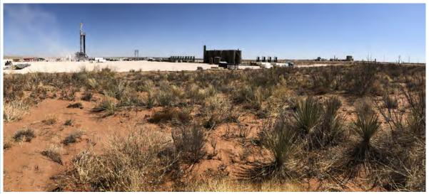
View east from showing the centralized tank battery pad on which the Colorado AST is planned. The well being drilled is one of several that will be stimulated with produced water stored in the AST..
