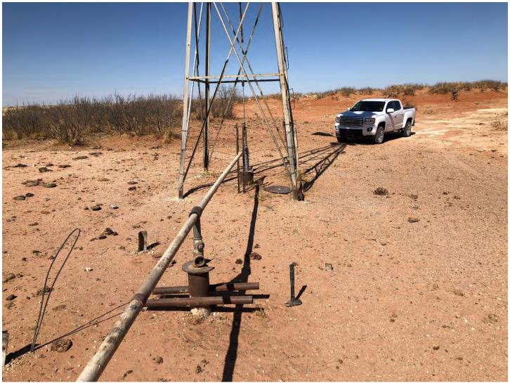
SP-5 — West Dublin Windmill that is a few feet north of SP-4. There is an abandoned casing in the foreground and the active windmill in the center of the image. Measuring depth to water in the windmill was no possible due to access and the sounder encountered dirt at a depth of about 120 feet.
