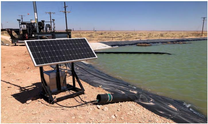
SP-1A Northwest corner of Gamma Ridge Containment #1 showing leak detection system
