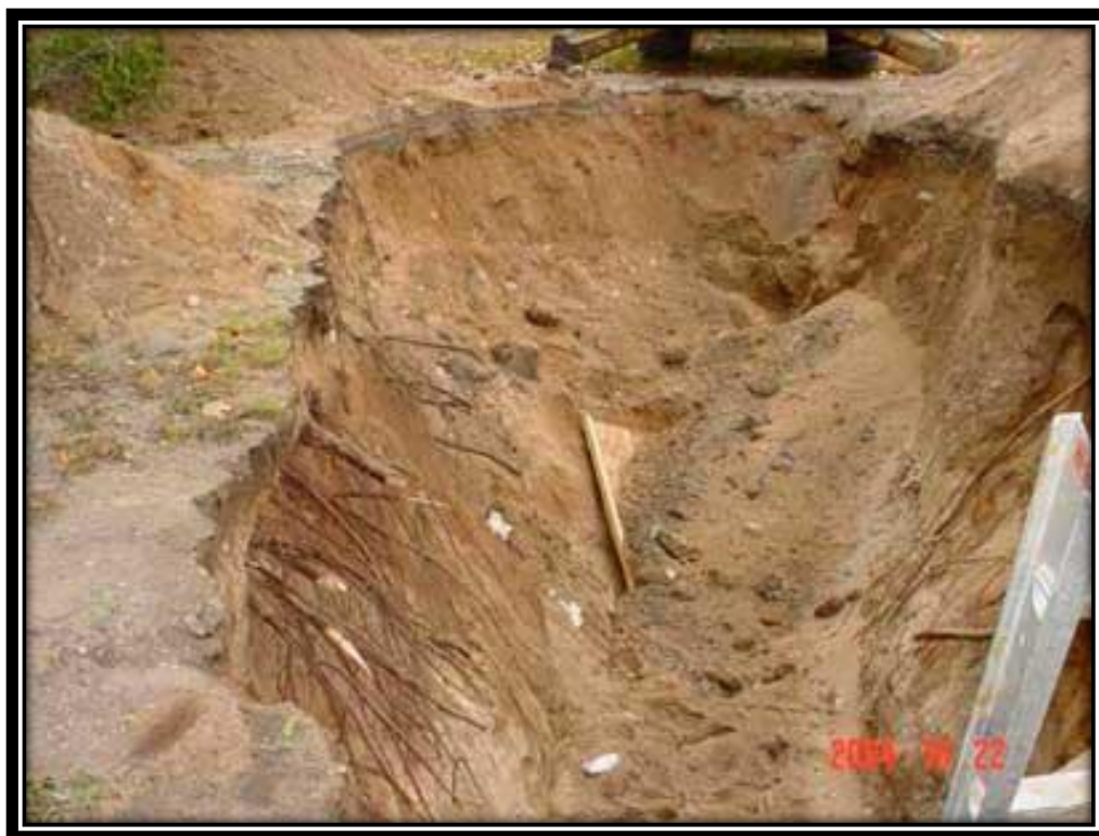
Figure 2. Example of trench collapse in loose sandy soil.
