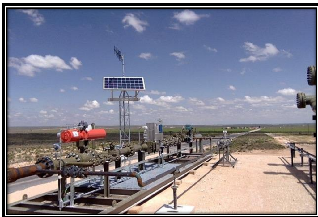
Figure 3. Typical layout of pig launcher and SCADA communications equipment.
