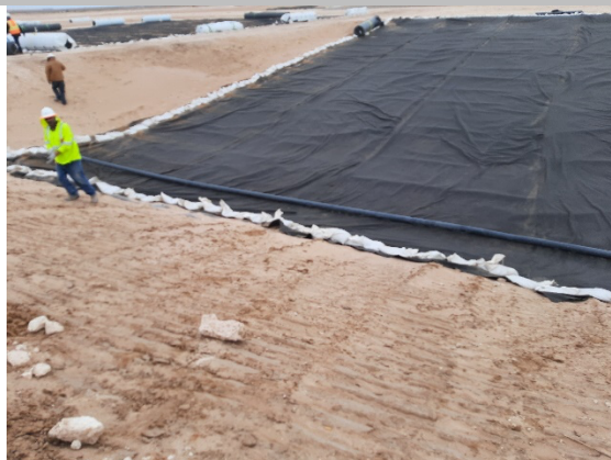
Filename: 20220330_095056 Installation crew placing additional sandbags in the truck wash.
