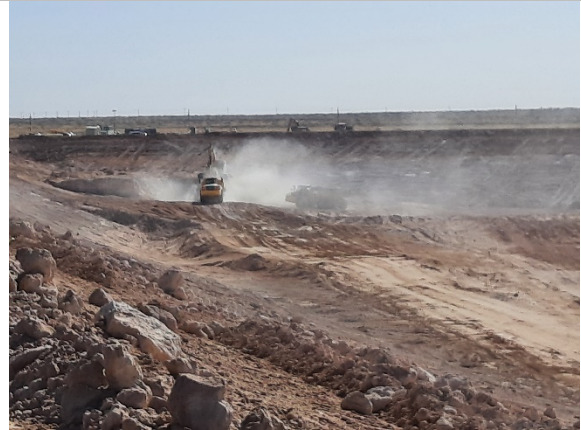
Filename: 20220406_092057 Excavators clearing material in the east section of Cell E1
