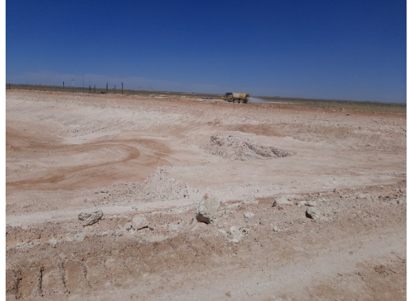
Filename: 20220405_113326 Water truck spreading water on the north berm of Cell E1
