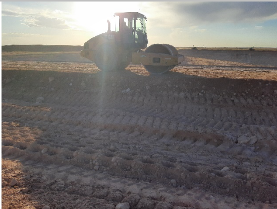
Filename: 20220404_181855 Smooth drum compacting material on the north berm of Cell E1
