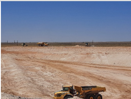
Filename: 20220406_133644 Haul truck placing material on the north berm of Cell E1
