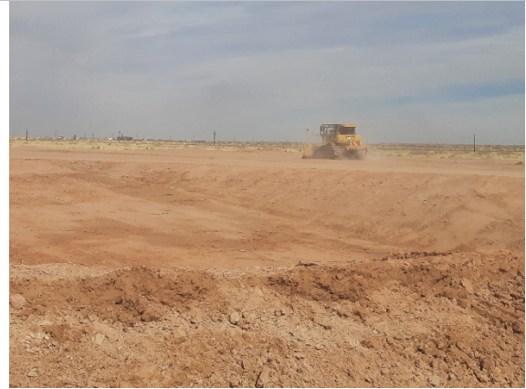
Filename: 20220223_135304 Dozer spreading material northeast of the truck wash area
