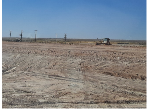
Filename: 20220402_160613 Dozer spreading material on the north berm of Cell E1
