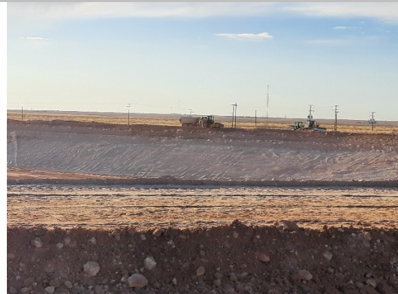
Filename: 20220404_182009 Water truck spreading water on the lift on the north berm of Cell E1
