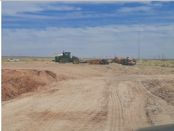
Filename: 20220223_135307 Tractor collecting excess cut material east of the truck wash pad
