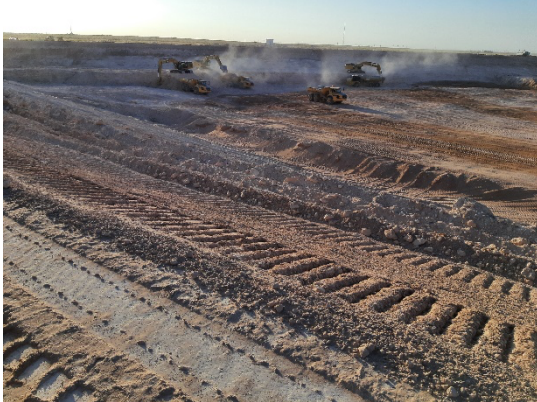
Filename: 20220404_073645 Excavators removing material from the east section of Cell E1
