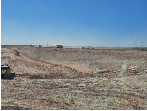
Filename: 20220402_160608 Haul trucks placing material for a lift on the north berm of Cell E1
