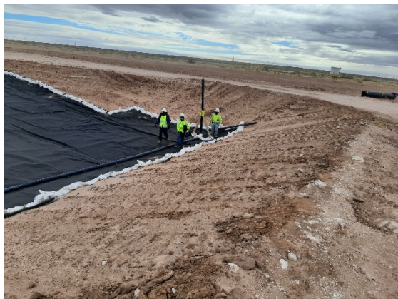
Filename: 20220330_095052 Description: Installation crew propping up pipe in truck wash
