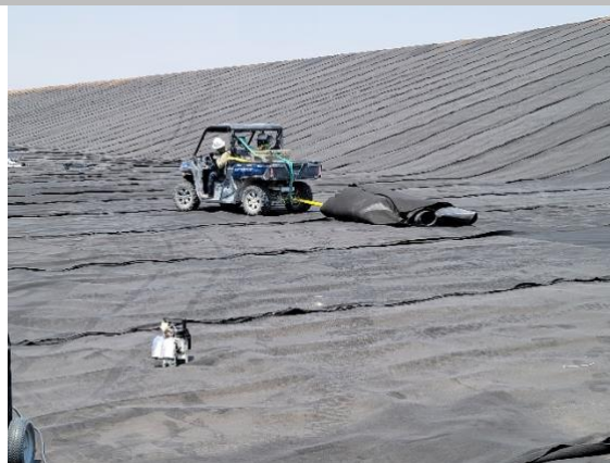
Filename: 20220519_112445 ATV moving geocomposite towards the trench in the floor of Cell E1
