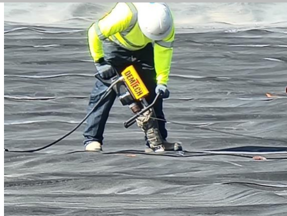
Filename: 20220528_085935 Welder extrusion welding a repair on the floor of the leachate pond
