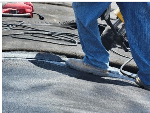
Filename: 20220517_113312 Installation crew extrusion welding replacement panel over P16
