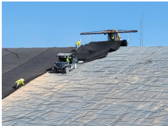
Filename: 20220513_092902 Installation crew using ATV to assist deploying geocomposite in Cell E1
