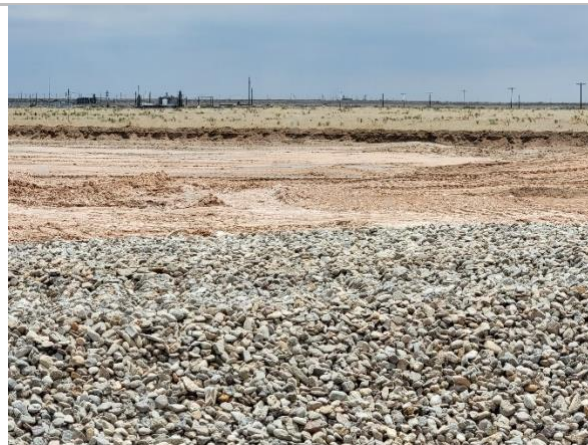
Filename: 20220602_134543 Rock for the sump being placed south of the cell ramp
