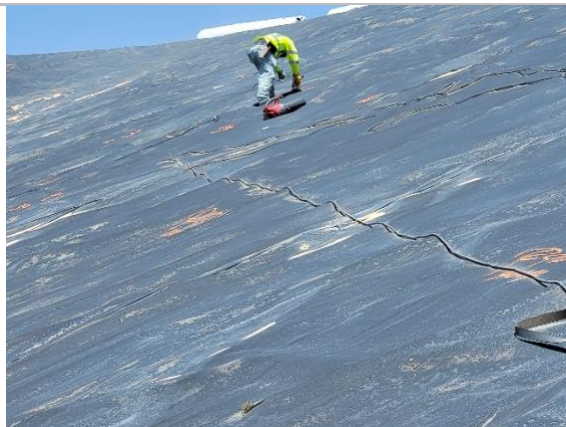
Filename: 20220512_140245 Installation crew cleaning and grinding a section to be repaired in the east slope
