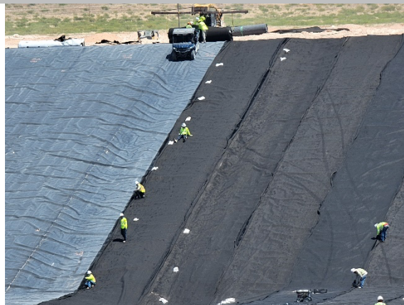
Filename: 20220506_135004 Installation crew securing exposed composite edge on the east slope
