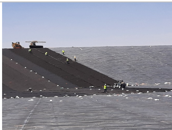
Filename: 20220502_144036 Installation crew deploying geocomposite on the north slope of Cell E1
