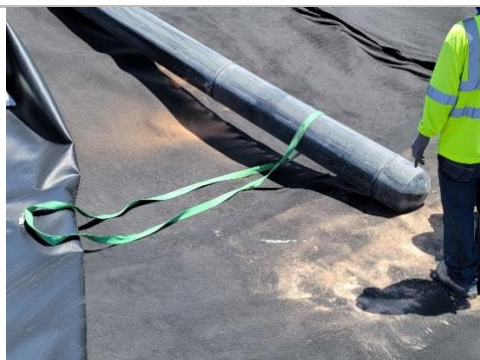
Filename: 20220527_113628 The 12" pipe being pulled into the sump of the leachate pond
