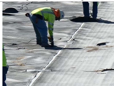
Filename: 20220512_082929 Installation crew leistering a patch on the floor of Cell E1
