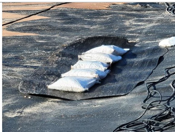
Filename: 20220603_073443 Installation crew placing sandbags on geomembrane for creating sand pillow
