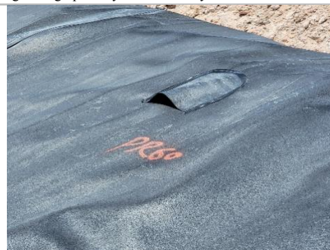
Filename: 20220528_120344 Cover fully welded over an air vent hole on the slope of the leachate pond
