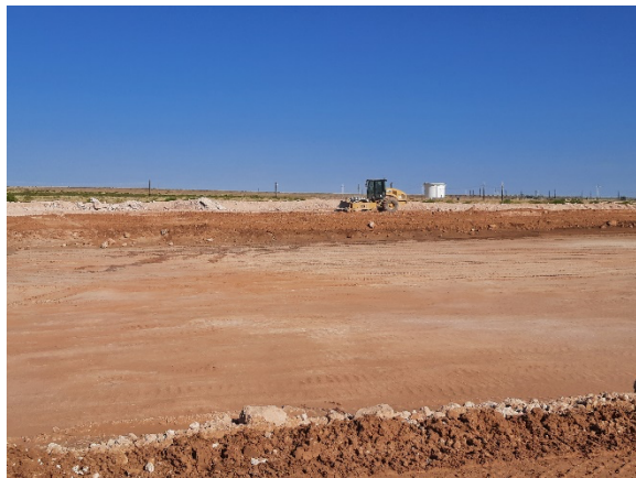
Filename: 20220426_165046 Compactor compacting lift on the east berm of the leachate pond
