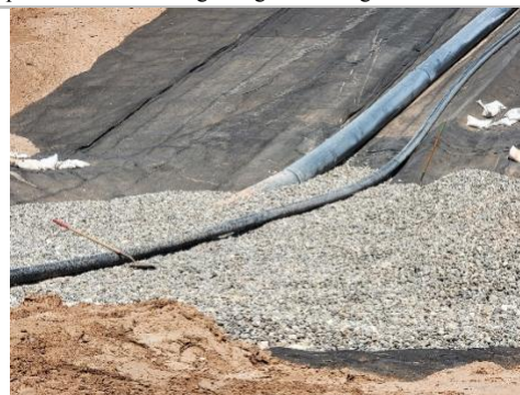
Filename: 20220527_145015 The 6" pipe being placed on top of the 2' of stone.
