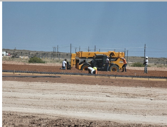
Filename: 20220505_150017 Forklift being used to assist the construction crew to create the forms
