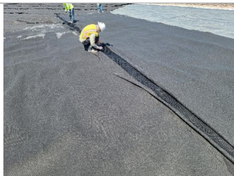
Filename: 20220513_145304 Installation crew using zip ties to connect geocomposite in Cell E1
