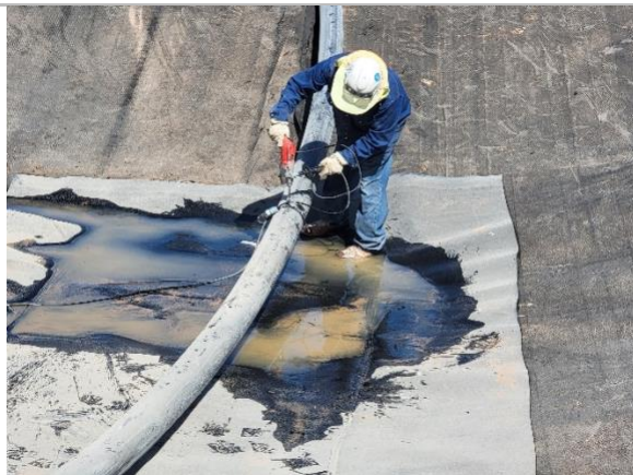
Filename: 20220526_094857 Pipe crew installing holes within the 6" pipe
