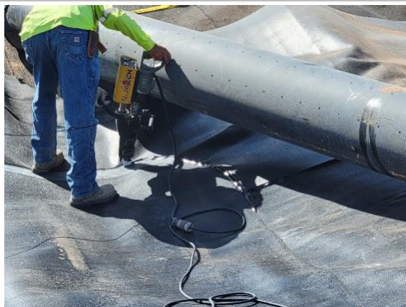
Filename: 20220526_090309 Installation crew welding the rub sheet within the sump of Cell E1
