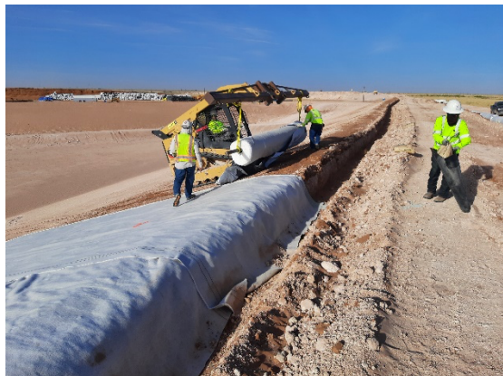
Filename: 20220423_074821 Installation crew deploying GCL on the north slope of Cell E1
