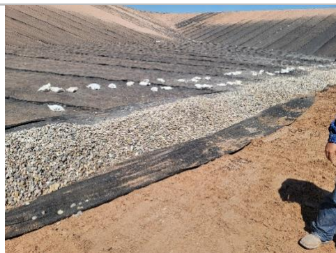
Filename: 20220526_150914 Stone being placed within the floor trench
