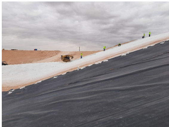
Filename: 20220425_081117 Installation crew deploying GCL on the north slope of Cell E1
