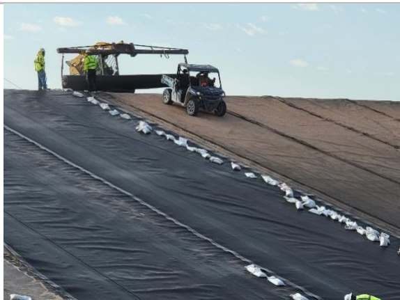
Filename: 20220510_075309 Installation crew using an ATV to deploy liner on the north slope of Cell E1
