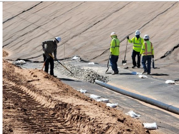
Filename: 20220525_152139 Installation crew spreading stone within the floor trench of Cell E1
