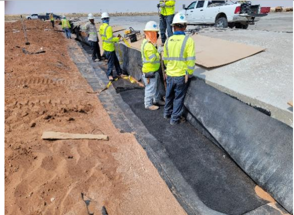
Filename: 20220601_101342 Installation crew lifting up primary liner system to be welded to the polylock
