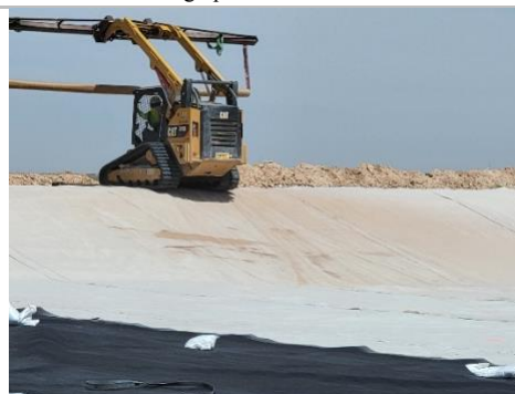
Filename: 20220520_110925 Skidsteer being used to deploy geomembrane in the leachate pond
