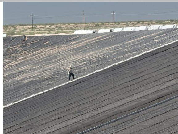
Filename: 20220510_171832 Installation crew anchoring the geomembrane with sandbags on the east slope
