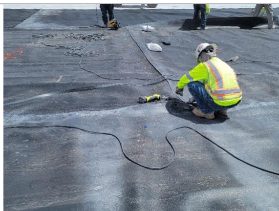
Filename: 20220520_110946 Installation crew setting up the air test within the leachate pond
