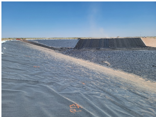
Filename: 20220506_134957 Installation crew deploying material on the east slope of Cell E1
