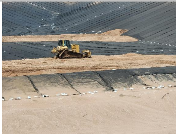
Filename: 20220524_134519 Dozer spreading material in the floor of Cell E1
