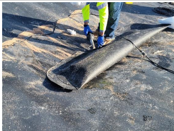
Filename: 20220603_072704 Installation crew leistering geomembrane to itself for sand pillow
