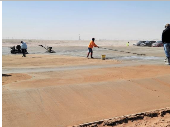
Filename: 20220521_092447 Concrete crew removing sand from concrete
