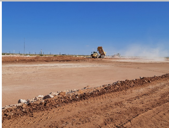
Filename: 20220426_165048 Haul truck transporting material in the east berm area of the leachate pond.
