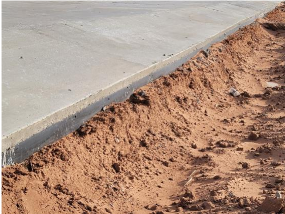
Filename: 20220601_073622 PC material being removed from the eastern edge to reveal polylock
