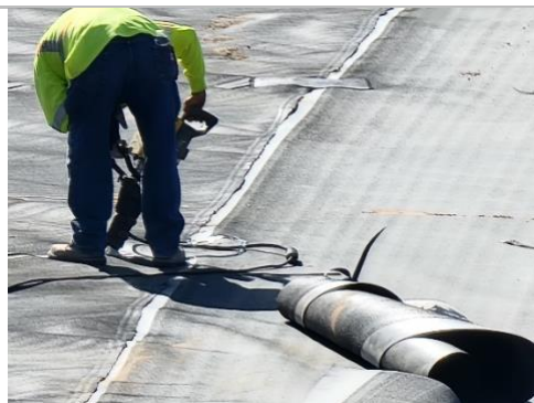
Filename: 20220512_082924 Extrusion welder welding a repair on the floor of Cell E1
