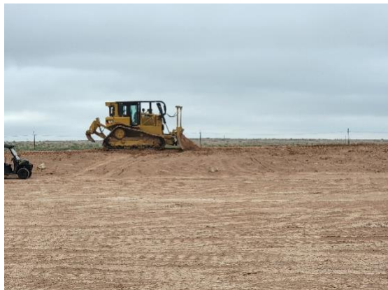
Filename: 20220602_085447 Dozer spreading excess material into the anchor trench of the leachate pond
