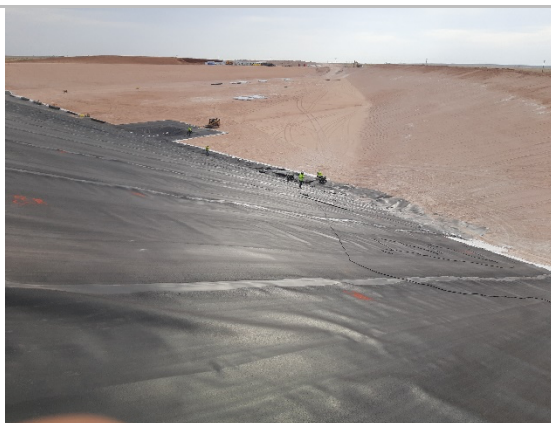
Filename: 20220419_182310 Installation crew air testing seams on the east berm north of the riser trench
