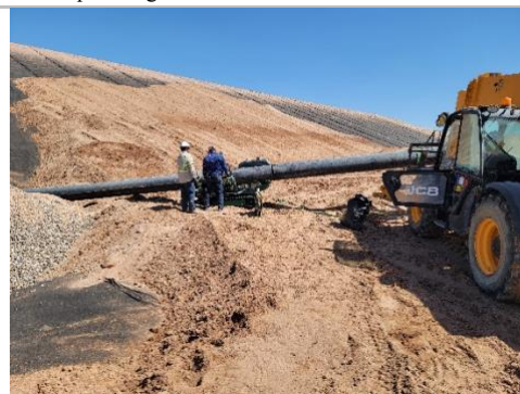
Filename: 20220526_152459 Pipe crew welding the straight 18" pipe end to the remainder of the 18" pipe
