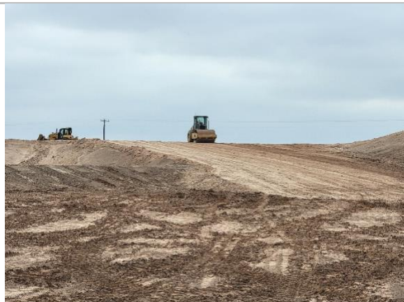
Filename: 20220602_132928 Smooth drum compacting material at the top of the cell ramp
