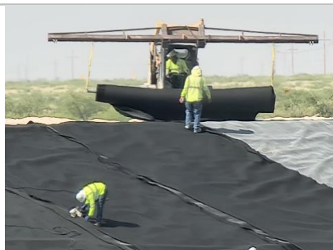
Filename: 20220518_154750 Composite being deployed in the northeast corner of Cell E1
