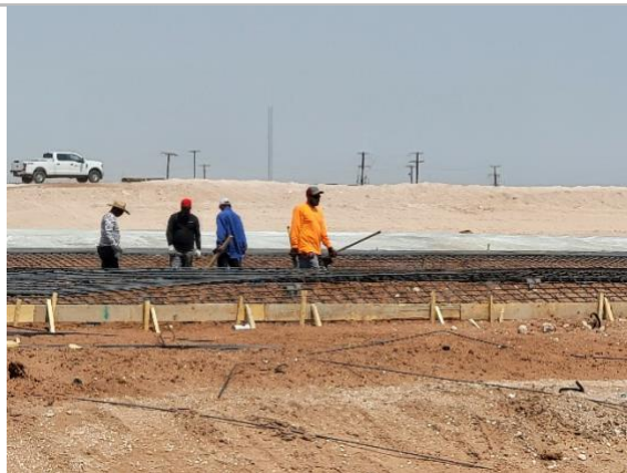
Filename: 20220518_110631 Construction crew preparing rebar forms in the east drying pad
