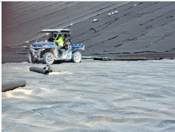
Filename: 20220514_100234 ATV being used to assist deploy the liner near the northeast corner of the floor.
