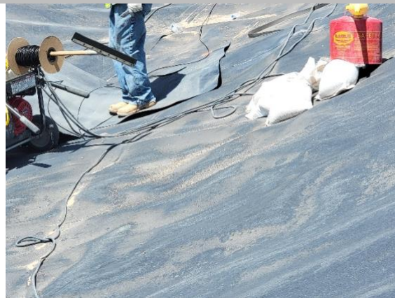
Filename: 20220512_140243 Installation crew cutting scrap liner to make a patch in the northeast corner
