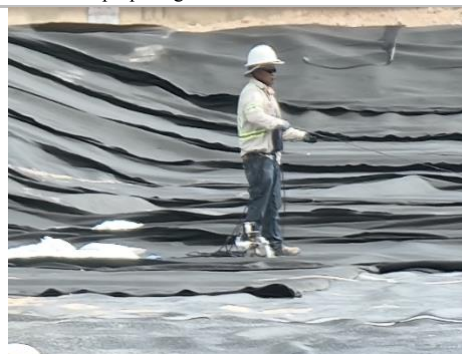
Filename: 20220524_144833 Installation crew using sewing machine to stitch geocomposite together in the pond
