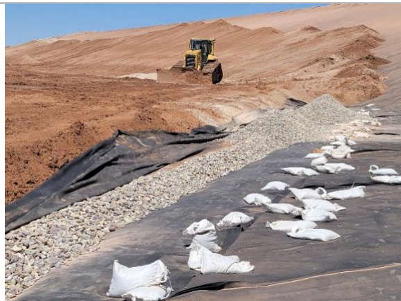
Filename: 20220526_104255 Dozer spreading material near the floor trench of Cell E1
