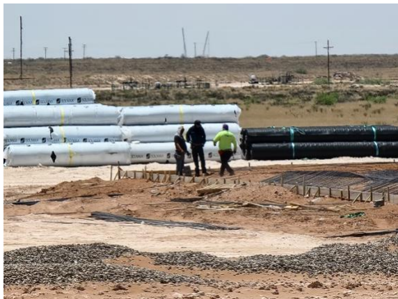
Filename: 20220517_122955 Construction crew working on rebar forms in the east drying pad
