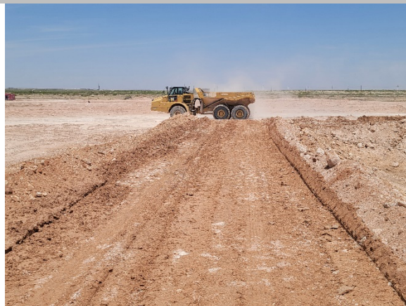
Filename: 20220503_124839 Haul truck transporting material to the north leachate berm
