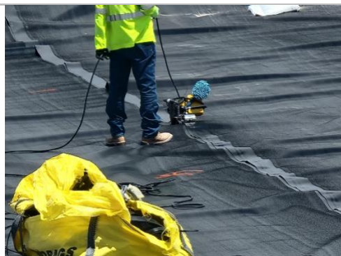
Filename: 20220523_142243 Installation crew fusion welding geomembrane overlap together
