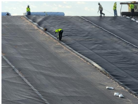
Filename: 20220511_075306 Welder cleaning and preparing overlap for welding on the east slope
