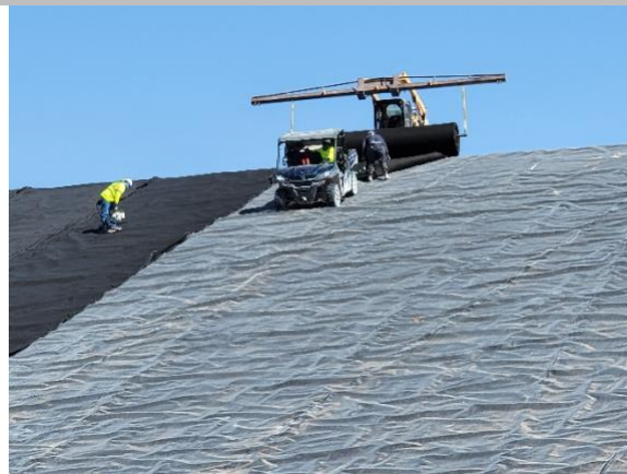
Filename: 20220514_100125 Installation crew using an ATV to assist pulling the liner on the north slope.
