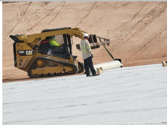
Filename: 20220523_083824 Installation crew spreading gcl on the floor of the leachate pond
