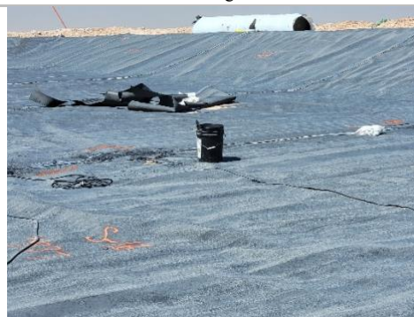
Filename: 20220521_102033 Installation crew placing water near a repair for vacuum box testing
