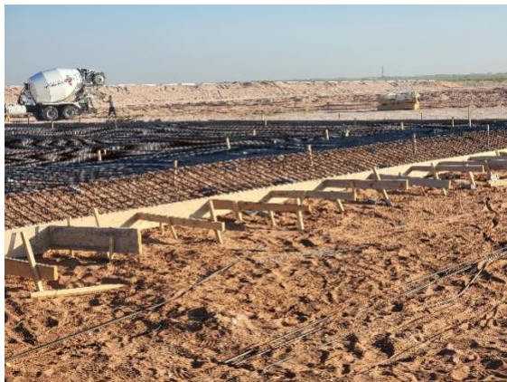
Filename: 20220514_071430 Rebar forms being made in the east drying pad
