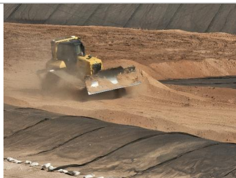
Filename: 20220521_092659 Dozer spreading material in the western part of cell e1
