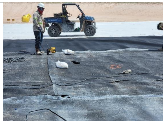
Filename: 20220520_082417 Repair in the riser trench being cleaned for extrusion welding
