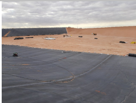
Filename: 20220425_081123 Installation crew preparing GCL to be deployed on the floor of Cell E1
