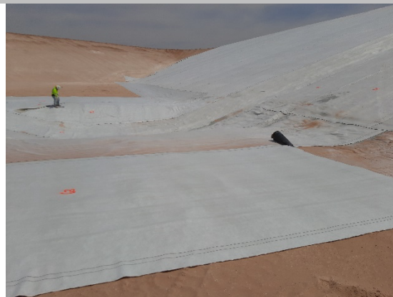
Filename: 20220419_123227 Installation Crew deploying GCL in the sump of Cell E1
