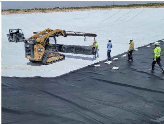
Filename: 20220523_142030 Installation crew deploying geomembrane on the floor of the leachate pond
