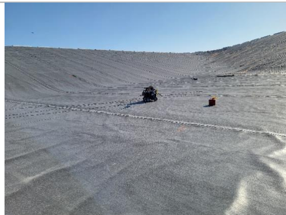
Filename: 20220512_080224 Mobile generator being used to power extrusion guns in the northeast corner
