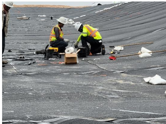
Filename: 20220524_080913 Installation crew vacuum box testing a repair in the leachate pond
