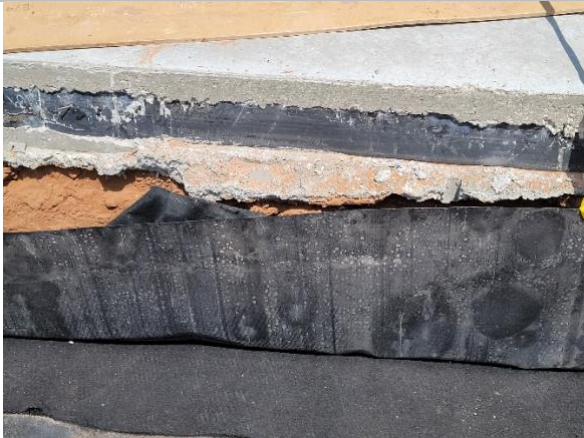
Filename: 20220601_102645 Excess concrete material that was removed from the west drying pad.
