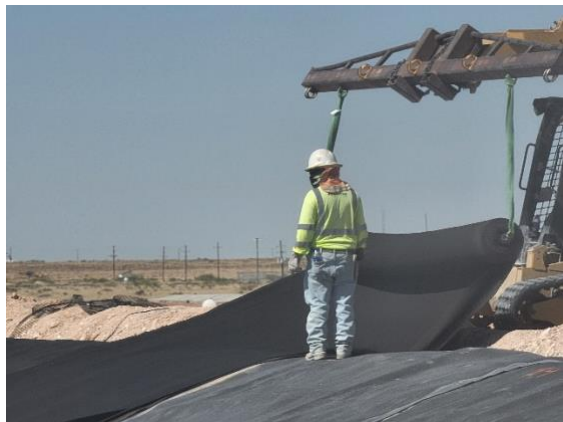
Filename: 20220525_094954 Installation crew deploying geocomposite in the leachate pond
