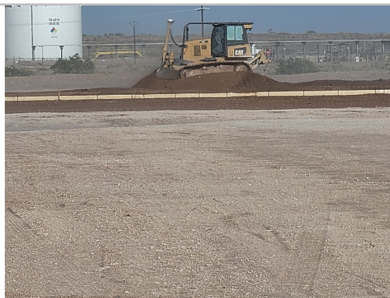
Filename: 20220428_173523 Dozer spreading PCL in the west drying pad.
