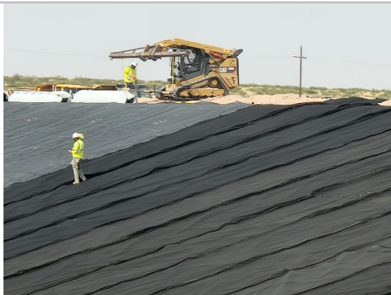
Filename: 20220506_161357 Skidsteer moving to transport geocomposite on the northeast corner of Cell E1
