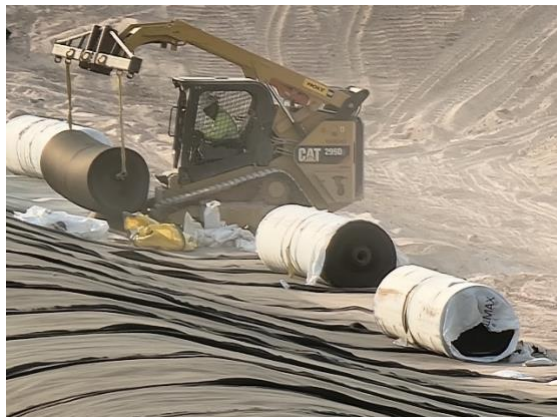
Filename: 20220519_074709 Skidsteer moving to the southern limit of Cell E1 to deploy geocomposite
