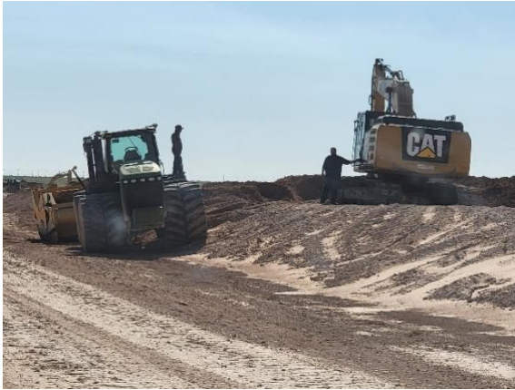
Filename: 20220606_085824 Excavator removing excess material from the ditch surrounding the Cell Berm
