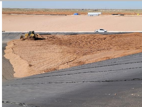
Filename: 20220520_084834 Dozer spreading material in the western part of Cell E1
