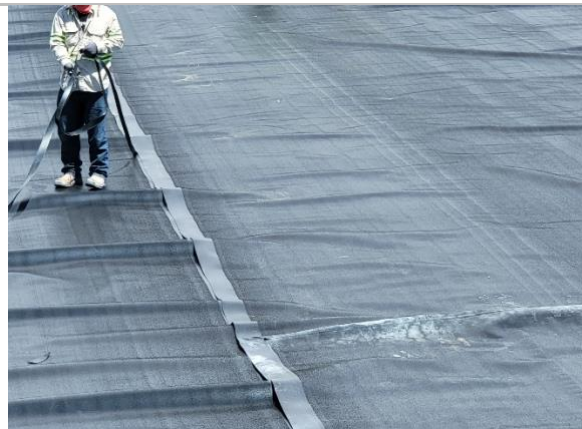
Filename: 20220523_142238 Installation crew preparing geomembrane overlap for welding
