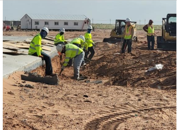
Filename: 20220601_083145 Installation crew removing excess PC material to reveal liner systems
