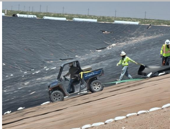
Filename: 20220511_133032 Installation crew using ATV to assist deploying liner on the east slope
