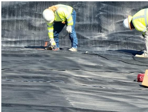
Filename: 20220528_085924 Installation crew cleaning overlap for extrusion welding
