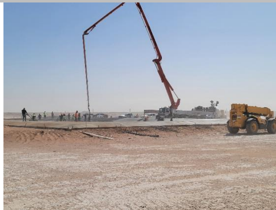
Filename: 20220521_092332 Concrete crew pouring and molding concrete in the east drying pad
