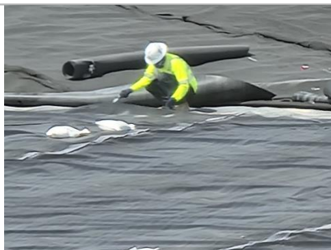
Filename: 20220516_150020 Installation crew cleaning overlap area in the center of the floor for welding
