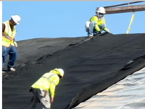
Filename: 20220513_093042 Installation crew pulling the geocomposite in line with adjacent panel
