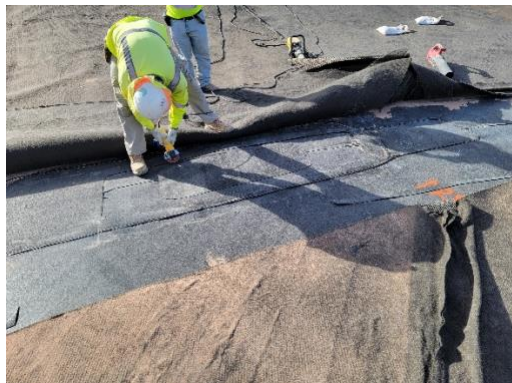
Filename: 20220521_075533 Installation crew cleaning repair for tracking destruct in Cell E1
