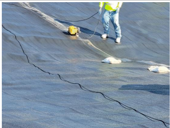
Filename: 20220527_082115 Installation crew fusion welding primary liner in the leachate pond
