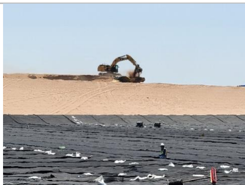
Filename: 20220519_133147 Excavator transporting PC onto a haul truck from the stockpile south of Cell E1
