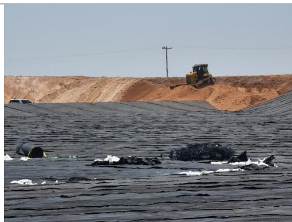
Filename: 20220519_133031 Dozer spread PC material at the western corner of Cell E1
