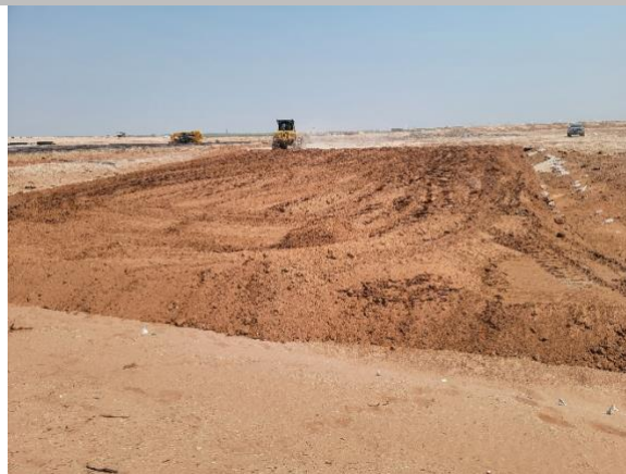
Filename: 20220518_110626 Dozer spreading drainage material in the truck wash
