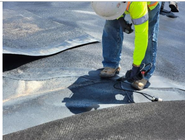
Filename: 20220517_112201 Installation crew leistering the repair panel over P16
