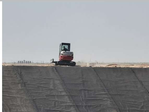
Filename: 20220517_161158 Excavator backfilling the anchor trench on the north slope of Cell E1
