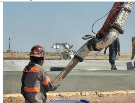
Filename: 20220514_154232 Construction crew clearing clog in the extended arm of the concrete mixer.
