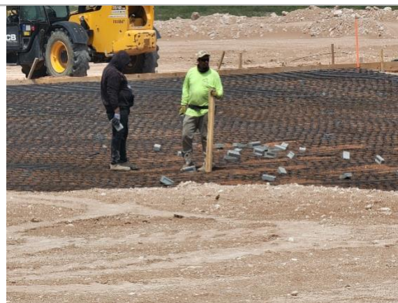
Filename: 20220524_143636 Construction crew preparing wooden form for use in the leachate pond
