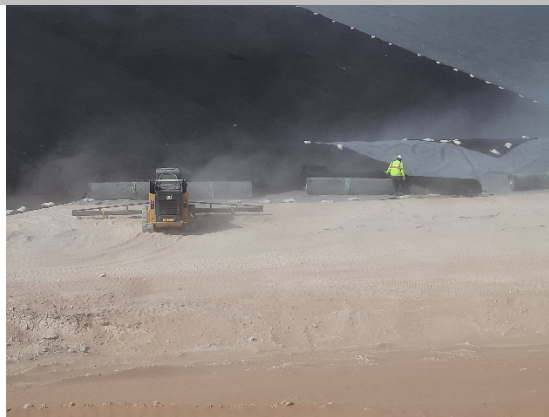
Filename: 20220429_161125 Installation crew placing material on the geocomposite placed in Cell E1
