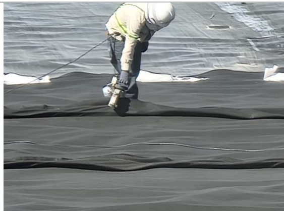
Filename: 20220517_161309 Installation crew stitching geocomposite together on the floor of Cell E1
