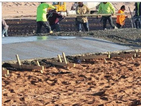
Filename: 20220514_071239 Concrete crew spreading material in the eastern part of the west drying pad.
