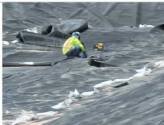
Filename: 20220516_150007 Welder cleaning the overlap for welding on the floor near the east slope
