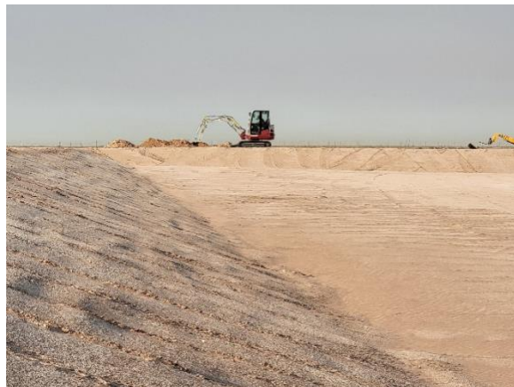
Filename: 20220518_074135 Excavator digging the anchor trench in the leachate pond berm
