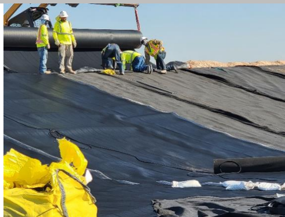
Filename: 20220527_082119 Installation crew deploying primary liner in the leachate pond
