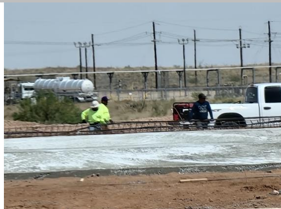
Filename: 20220516_150052 Construction crew adjusting rebar to build the forms in the east drying pad
