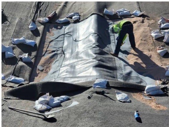
Filename: 20220520_082417 Repair in the riser trench being cleaned for extrusion welding
