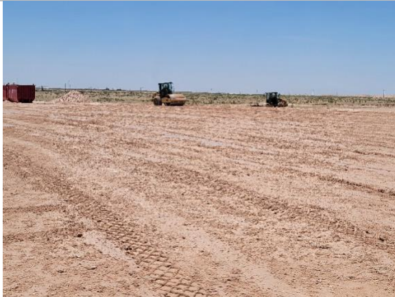
Filename: 20220606_123057 Smooth drum preparing to compact Caliche Road
