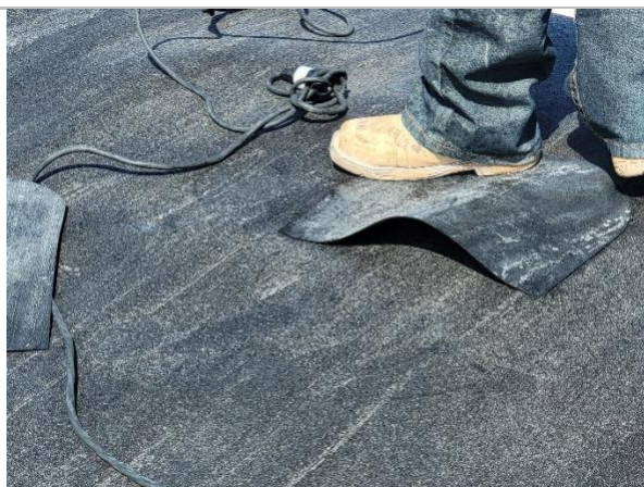
Filename: 20220528_091422 Installation crew preparing cover of air vent for welding
