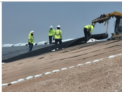
Filename: 20220511_133034 Installation crew straightening out the liner on the east slope of Cell E1
