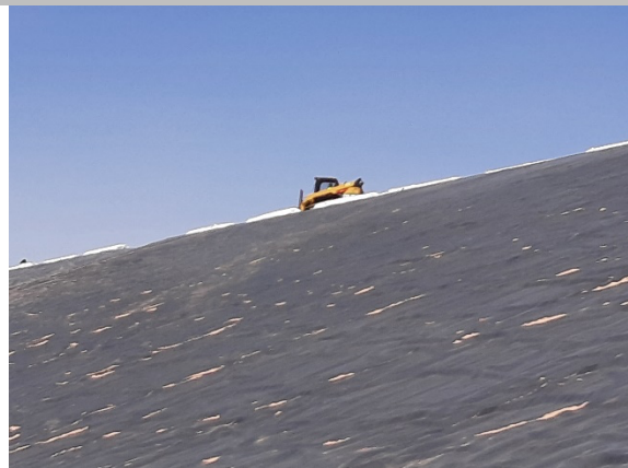
Filename: 20220502_144033 Skidsteer being used to pull geocomposite for deployment
