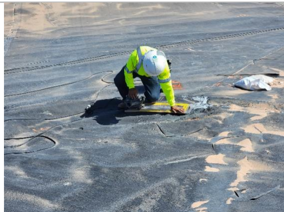
Filename: 20220513_094938 Installation crew vacuum boxing repairs within the floor of Cell E1
