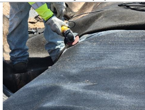
Filename: 20220517_113316 Installation crew gridding overlap of the replacement panel and P16
