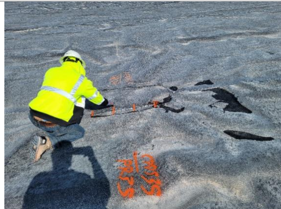
Filename: 20220511_091047 Installation crew QC cutting marked destruct in the northeast part of Cell E1
