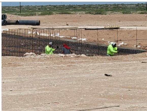
Filename: 20220524_143630 Construction crew placing rebar forms vertically in the truck wash
