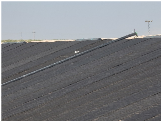
Filename: 20220509_155046 12" pipe being placed within the east trench riser
