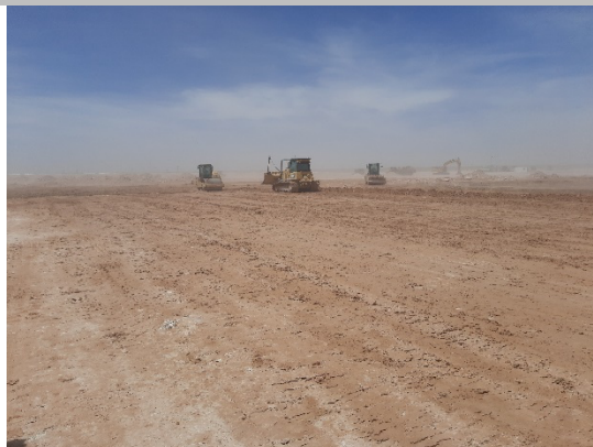
Filename: 20220423_132405 Dozer spreading material in the east berm area of the leachate pond.
