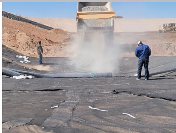
Filename: 20220526_094337 Stone being transported to the sump of Cell E1
