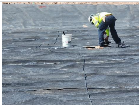
Filename: 20220528_100751 Installation crew doing vacuum box testing on the repairs in the leachate pond
