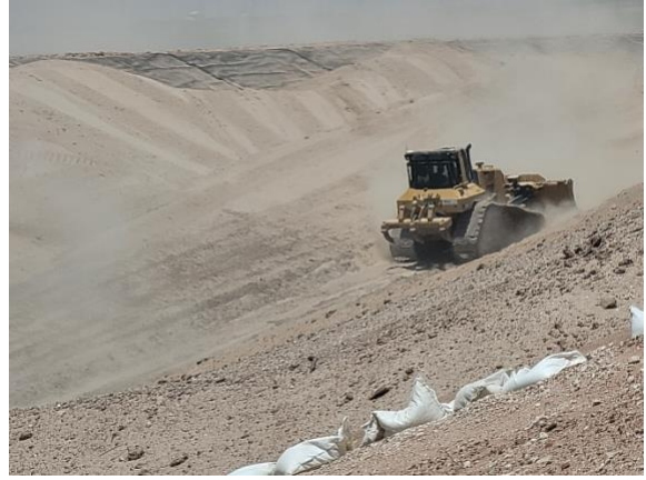
Filename: 20220531_132237 Dozer spreading material up the northeast corner of Cell E1
