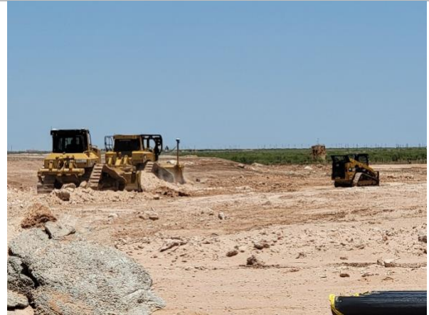
Filename: 20220606_123101 Dozers spreading material on the Caliche Road
