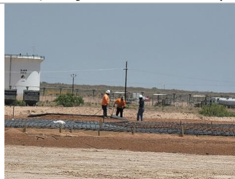
Filename: 20220511_133043 Construction crew preparing steel forms in the northern part of the east drying pad
