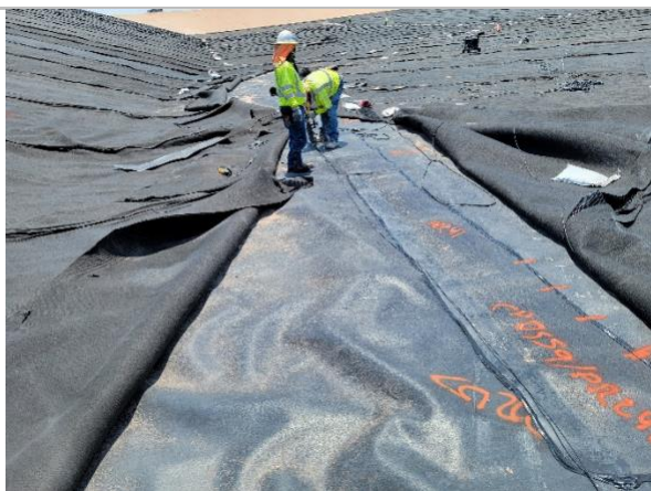
Filename: 20220519_133016 Installation crew welding a cap over the failed seam in Cell E1
