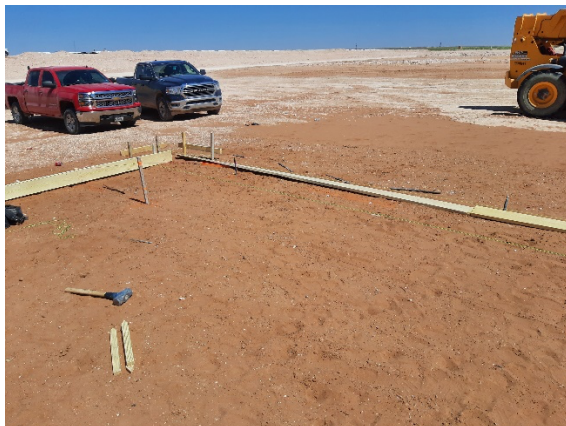
Filename: 20220428_110447 Forms getting setup in the northwest corner of the west drying pad.
