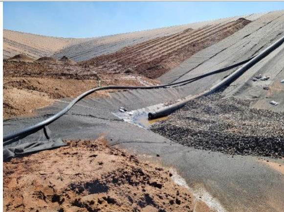
Filename: 20220527_090909 6" pipe being removed from the sump in order for the 2' of stone to be placed.
