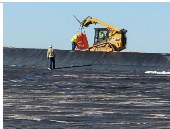
Filename: 20220603_074432 Installation crew transporting sandbags to the leachate pond for the sand pillows.
