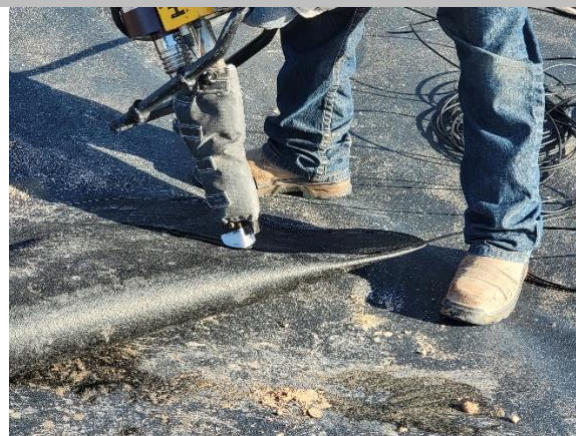
Filename: 20220603_073036 Installation crew extrusion welding sand pillow in leachate pond
