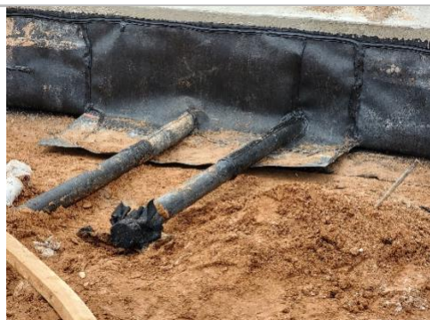
Filename: 20220602_144603 Boot installed on the east drying pad
