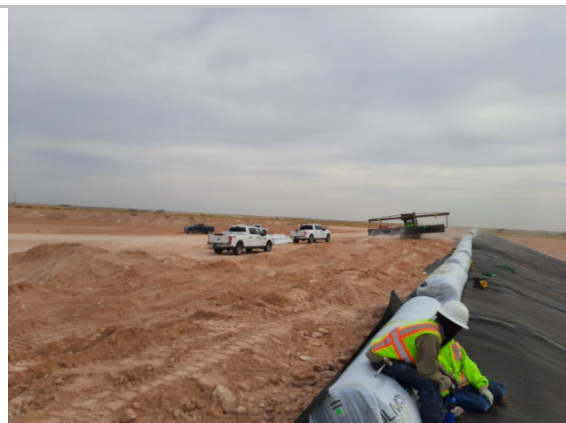
Filename: 20220419_175720 Skidsteer transporting liner on the east berm of Cell E1
