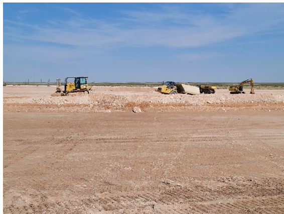
Filename: 20220503_093134 Dozer spreading material on the north leachate berm
