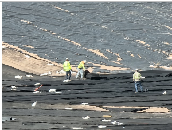
Filename: 20220506_161408 Installation crew pulling geocomposite into place on the floor of Cell E1
