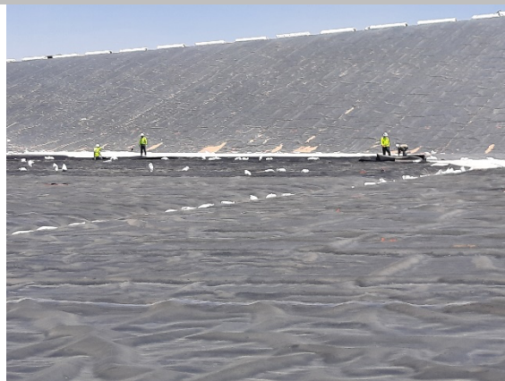
Filename: 20220428_134344 Installation crew deploying geomembrane near the east toe of the slope of Cell E1
