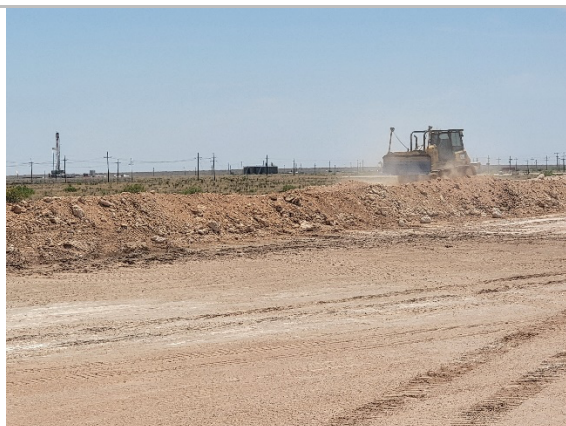
Filename: 20220503_124834 Dozer spreading material on the east leachate berm
