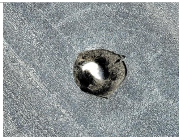
Filename: 20220528_091623 Hole cutting through primary and secondary liner to the GCL for the air vent
