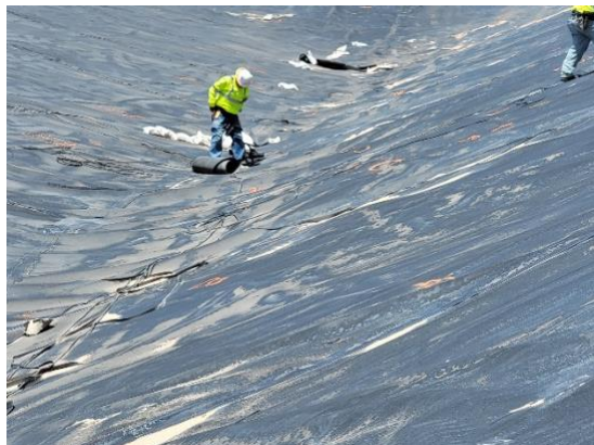
Filename: 20220512_140241 Welder preparing patch to be welded in the northeast corner
