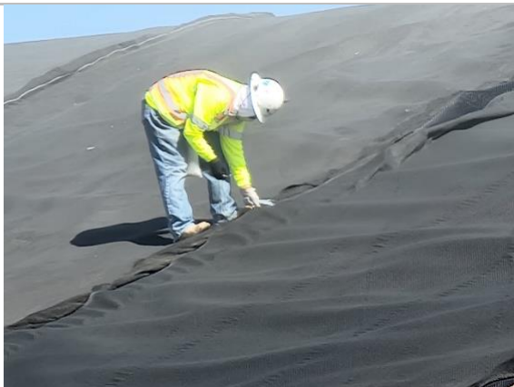
Filename: 20220513_093128 Installation crew opening overlap of panels for zip ties on the north slope of Cell E1
