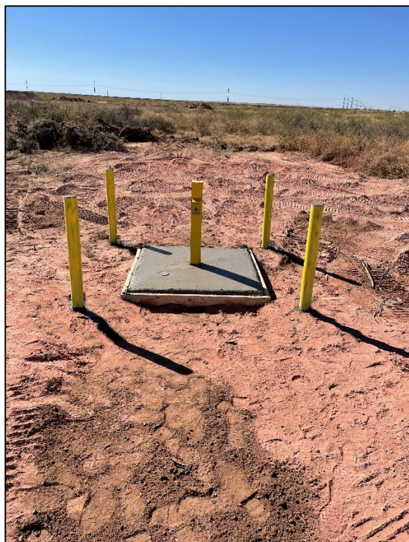
Well LLC VZ-4 Surface completion.
