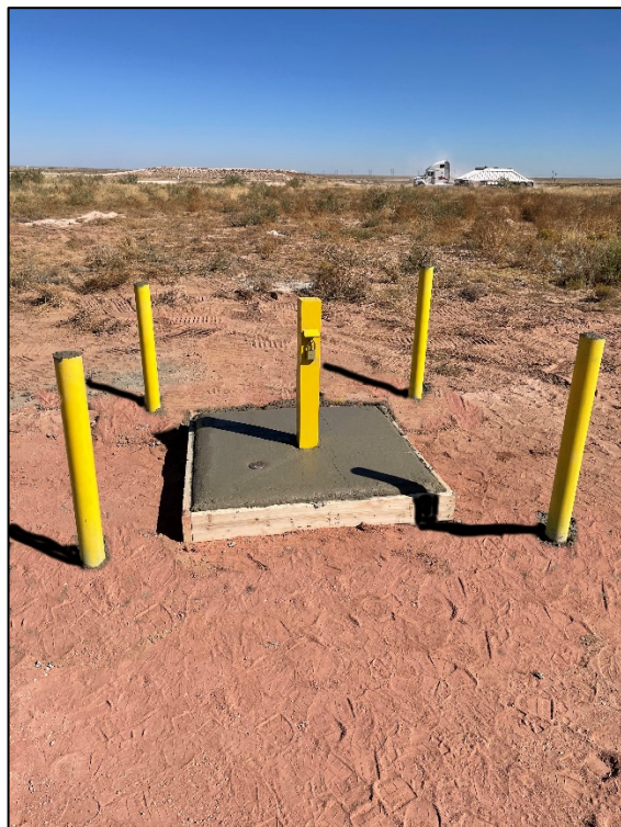
Well LLC VZ-3 Surface completion.
