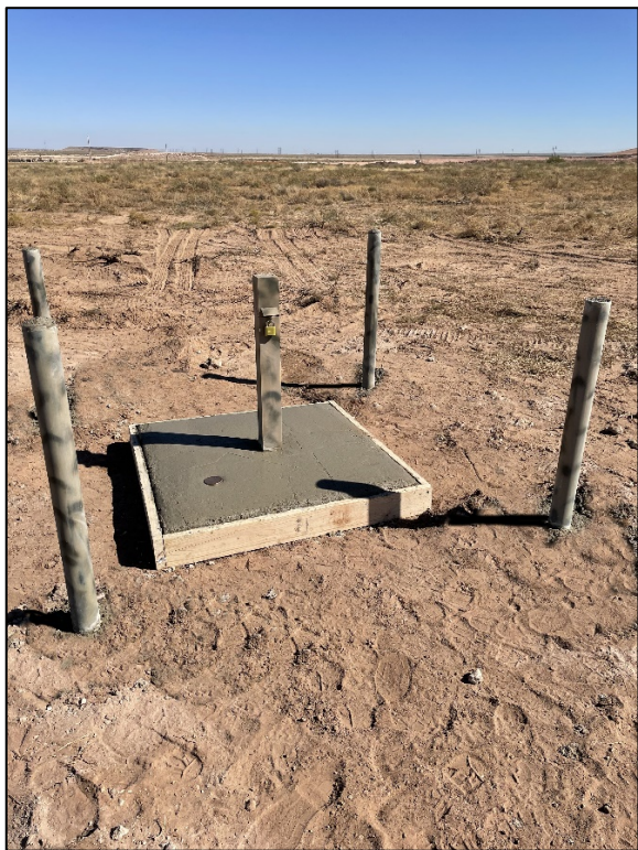
Well LLC VZ-1 Surface completion.
