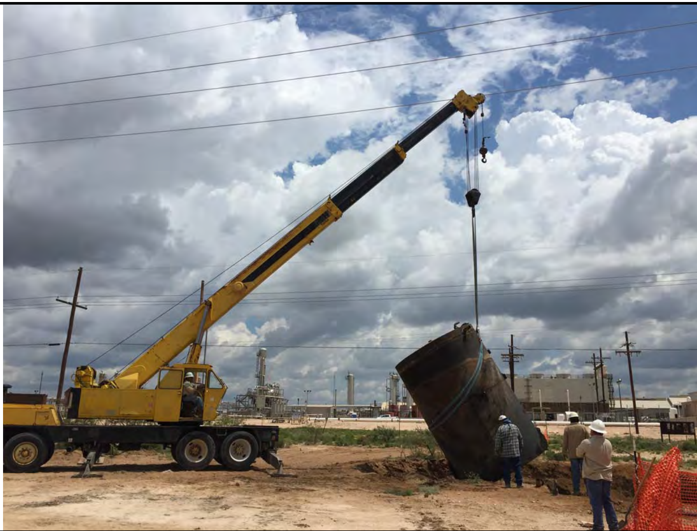
Photo 4: View of the removal of the northern field scrubber BGT, facing east.
