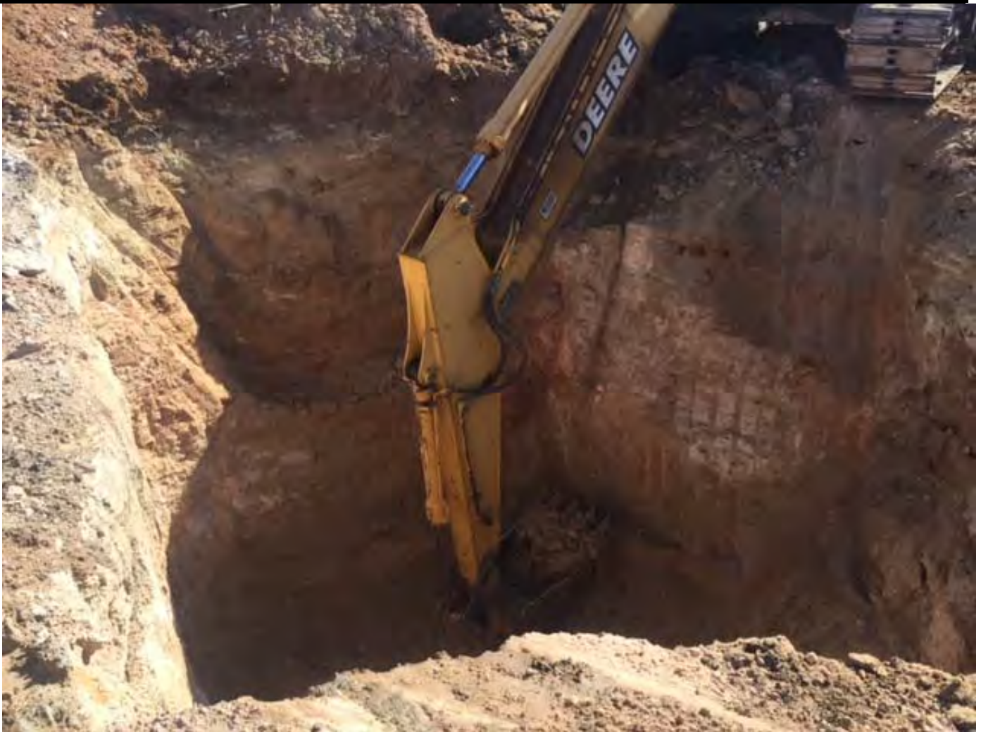
Photo 13: View of excavation of affected soil adjacent to the southern BGT's former location, facing east.
