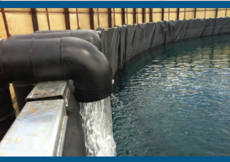
Tank Tech uses High Density Polyethylene for all mechanical applications.
