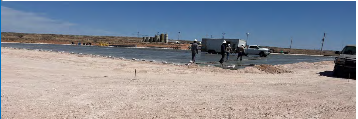
Placement of liner for secondary containment of OXY Lost Tank AST Containment on the existing OXY USA pad.
