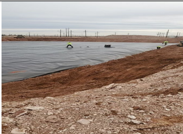
Photo 2: View of liner installation.
