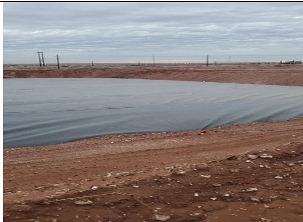
Photo 1: View of liner installation.
