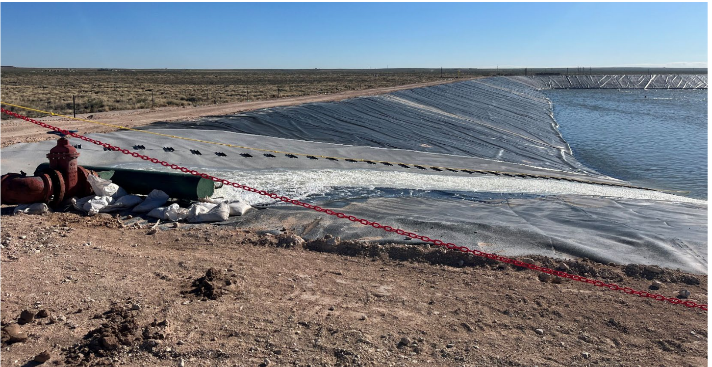
SP-4 Filling the Lois Lane Rule 34 Containment to permit produced water use for hydraulic stimulation soon after construction completion. Image taken October 26, 2022.
