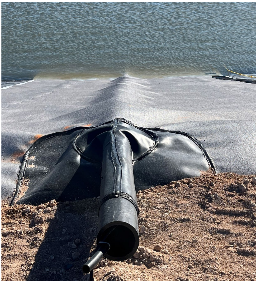
SP-5 Leak detection monitoring pipe on west side of containment (10/26/22)
