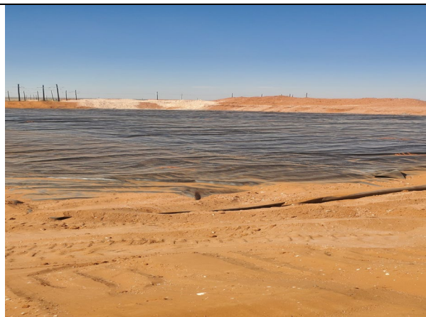
Photo 2: Overview of final liner installation.
