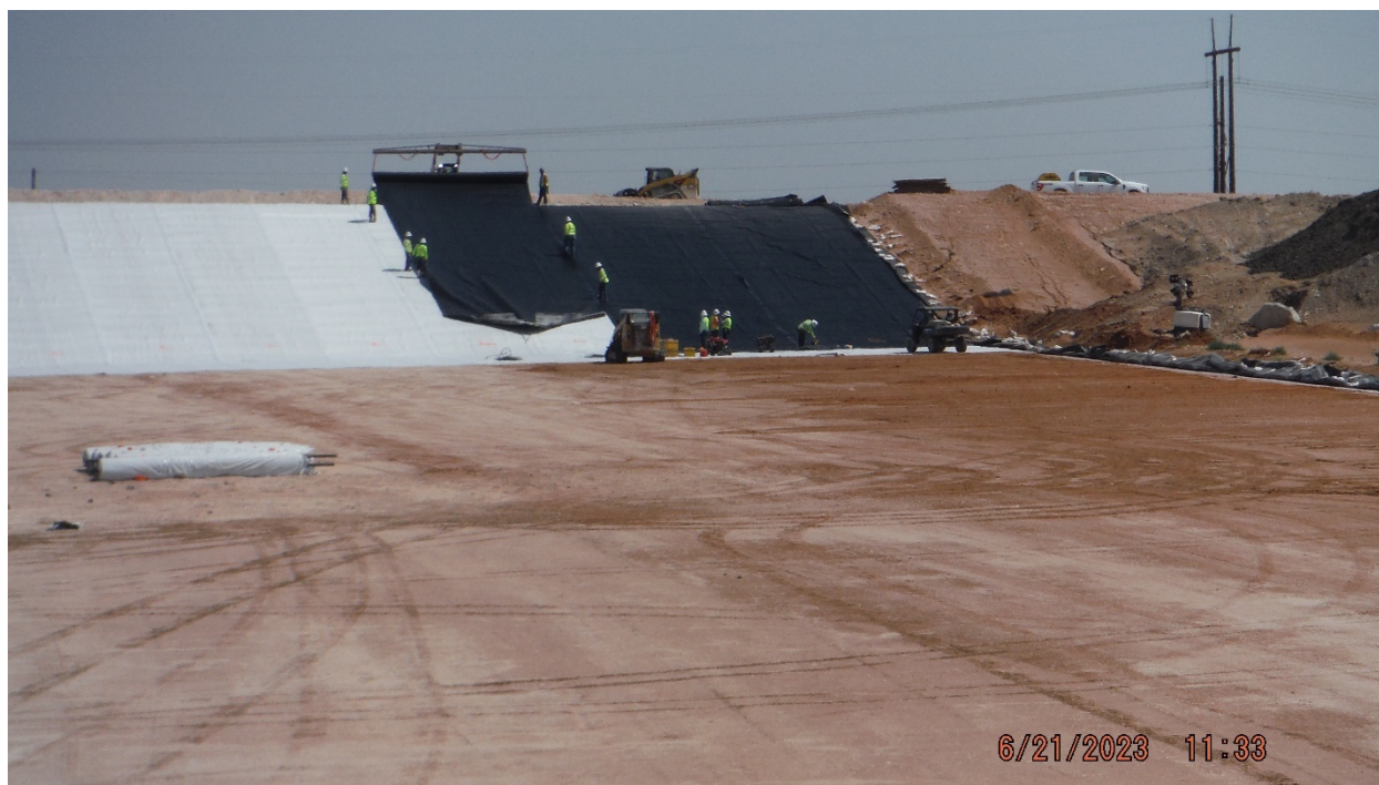
2023-06-21: Secondary HDPE Deployment on Slope
