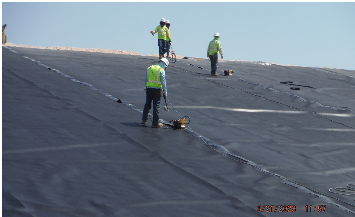
2023-06-21: Welding of Secondary HDPE
