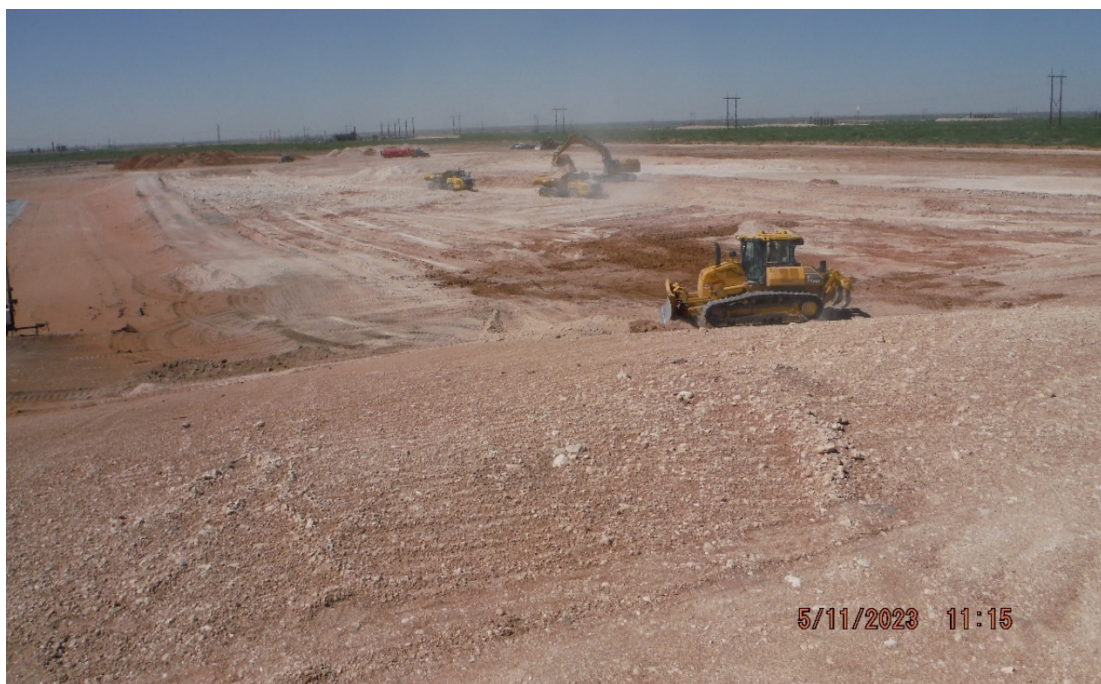
2023-05-11 Excavation of Cell 5AB.
