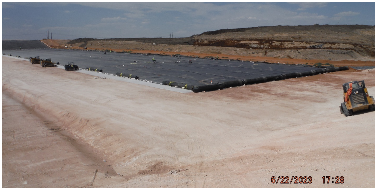
2023-06-22: Secondary HDPE Deployment on Floor
