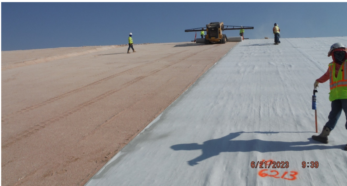
2023-06-21: GCL Deployment on Slope
