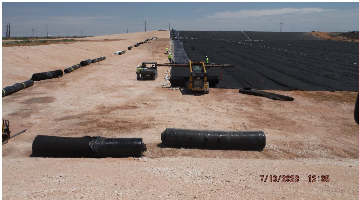
2023-07-10: Deployment of Geocomposite
