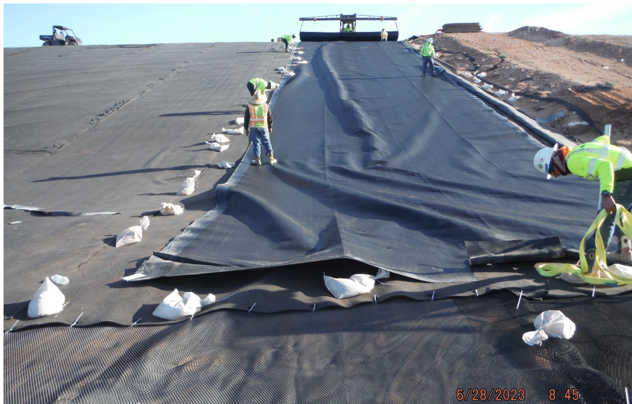
2023-06-28: Primary HDPE Deployment on Slope
