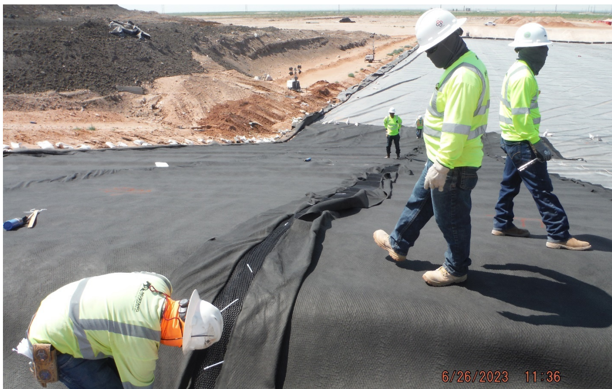
2023-06-26: Geocomposite Deployment on Slope
