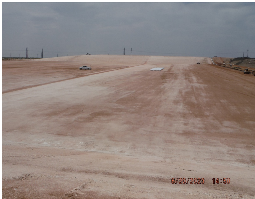
2023-06-20: Completed Subgrade
