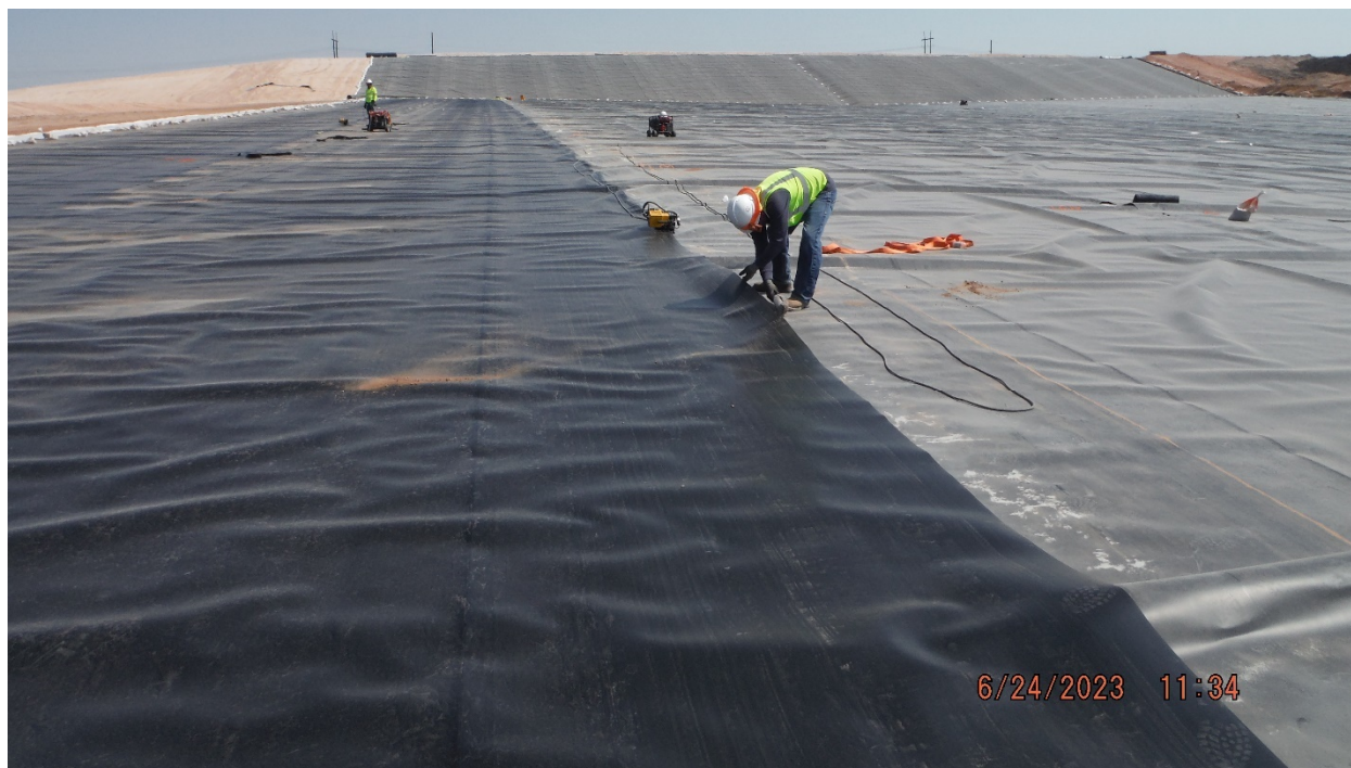
2023-06-24: Secondary HDPE Welding on Floor
