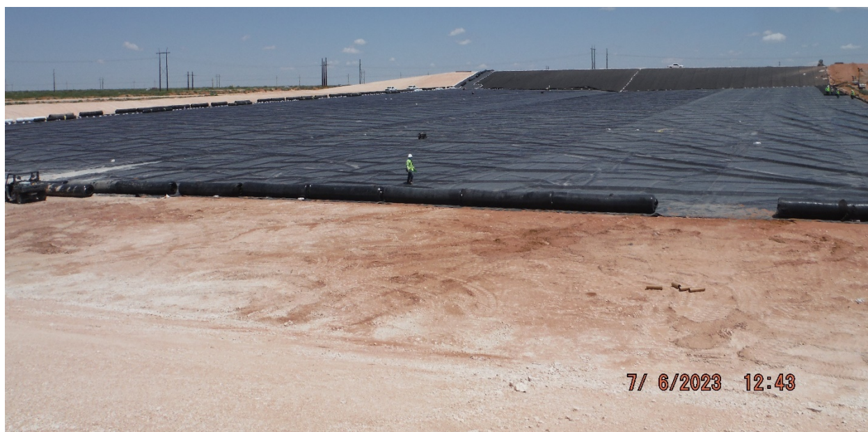
2023-07-06: Completed Deployment of Primary HDPE
