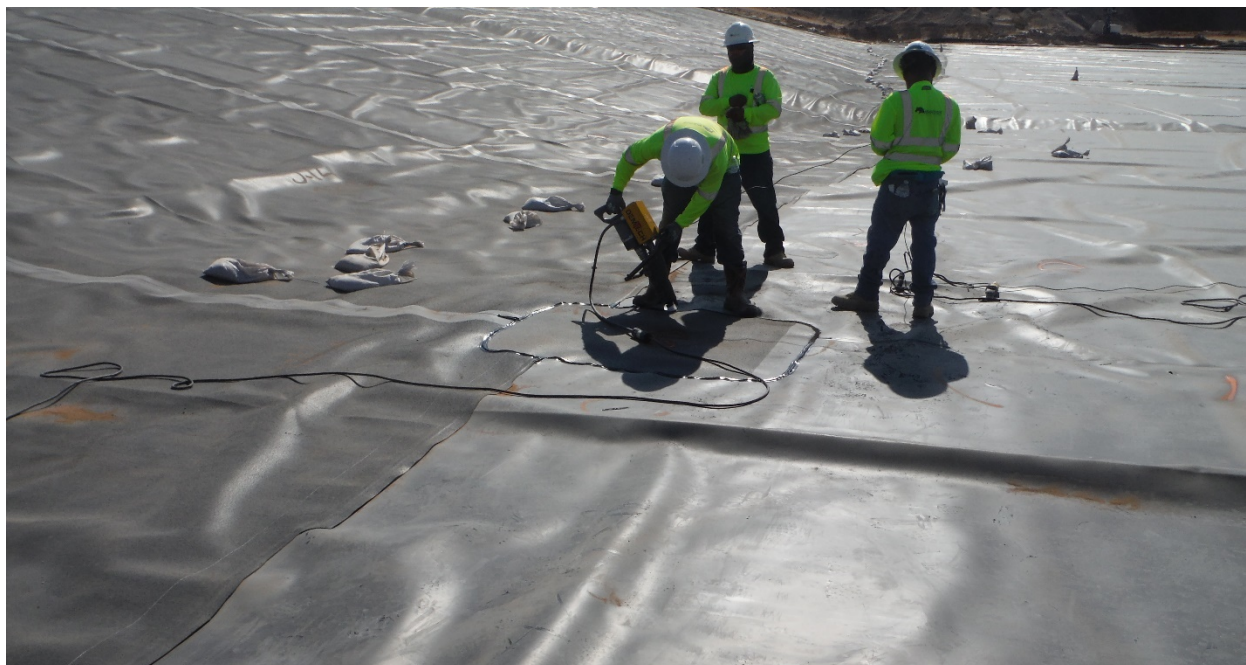
2023-06-26: Repair of Secondary HDPE at T-intersection
