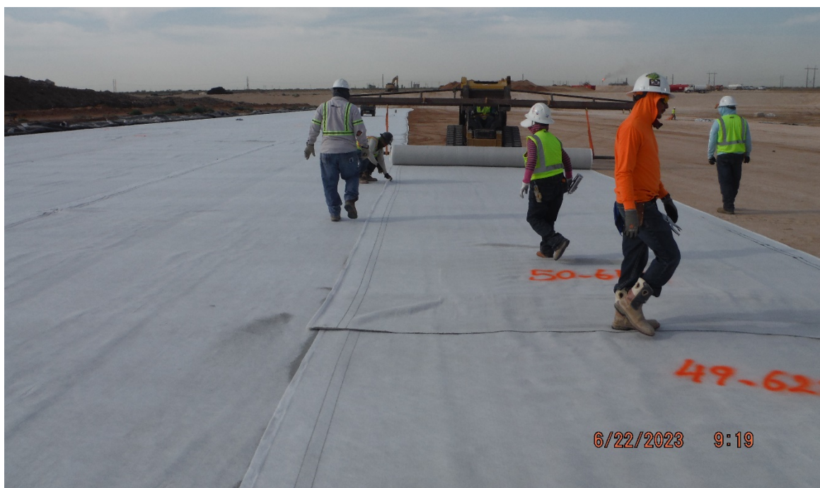
2023-06-22: GCL Deployment on Floor
