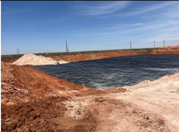
Photo 2: Overview of liner installation.
