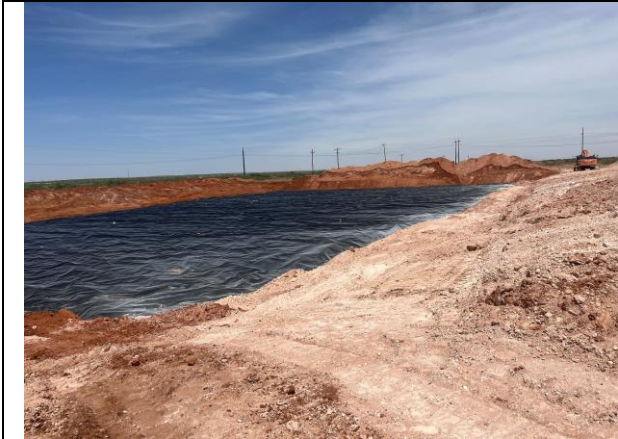
Photo 1: Overview of liner installation.
