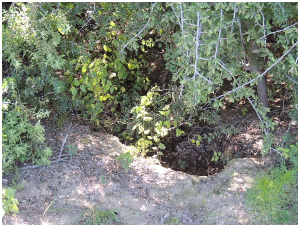
SURFACE DEPRESSION WITH DRAINAGE HOLE, 564669E, 3543067N
