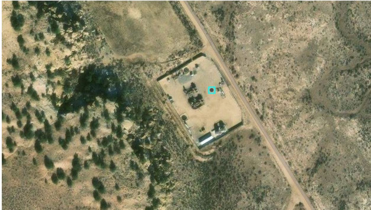
Figure 1.5 Otero Compressor Station
