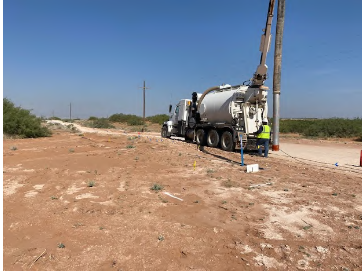
Photograph 5: View of hydrovac deploying to spot lines in area.
