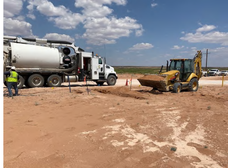
Photograph 6: View of hydrovac spots being backfilled.
