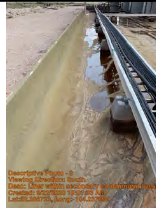
Liner within secondary containment (west wall)
