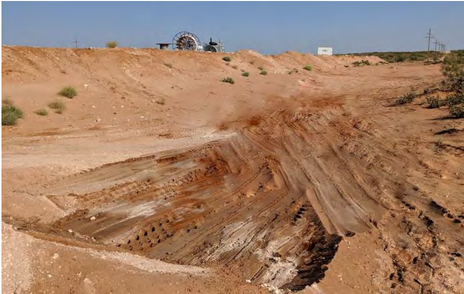
Figure 2: Restoration of release area as a right-of-way access to the eastern berm of the Wool Head A Pad for maintenance operations. The pinkish-white soil is caliche. GPS: 32.4572861 N, 103.5875600 W. Date/Time: 2020-09-18 09:09:28.
