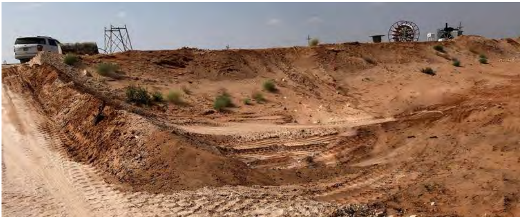
Figure 3: Reuse of source material for beneficial use as lease road berm material to prevent unauthorized access to right-of-way along east side of production pad.
