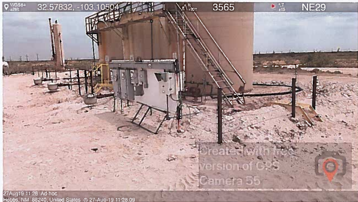
Area excavated with new installed berm
