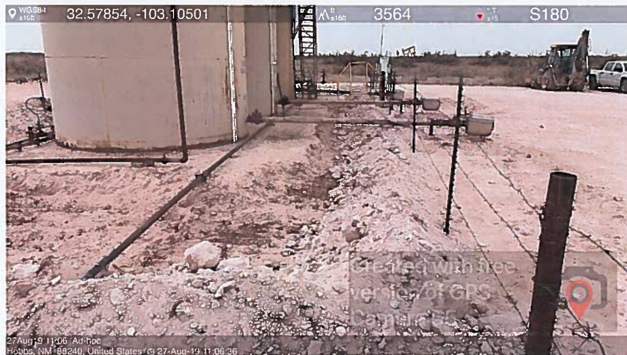
Area excavated with new installed berm
